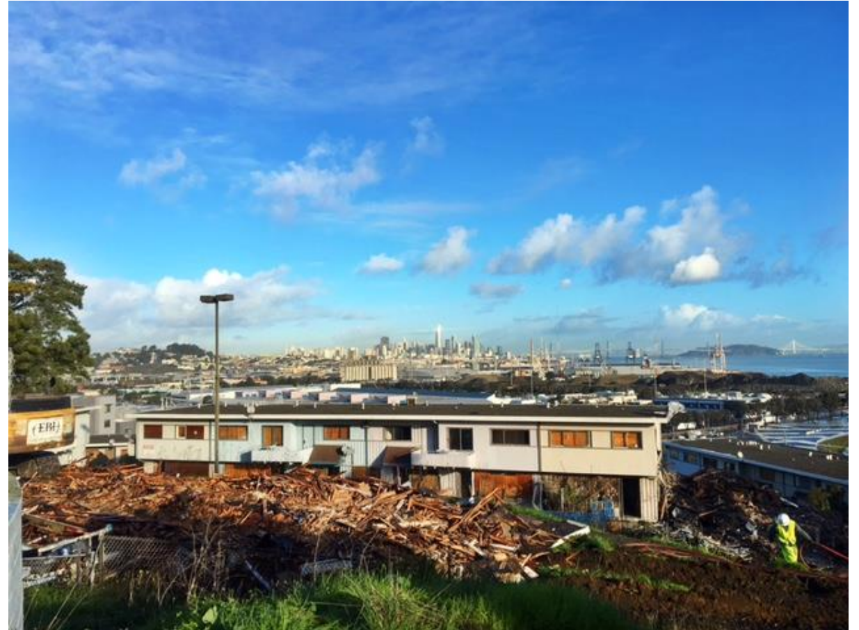
Site preparation activities in Phase 3 (2018).
