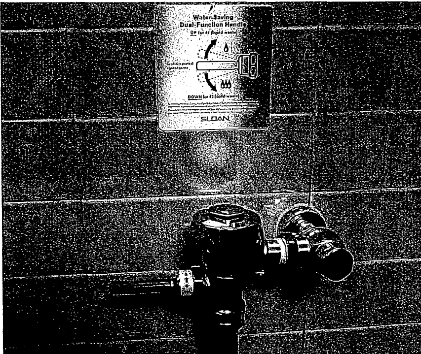
Dual flush toilets contribute to indoor water use reduction
