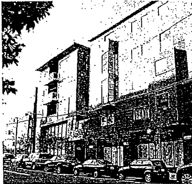
Examples of significant breaks
