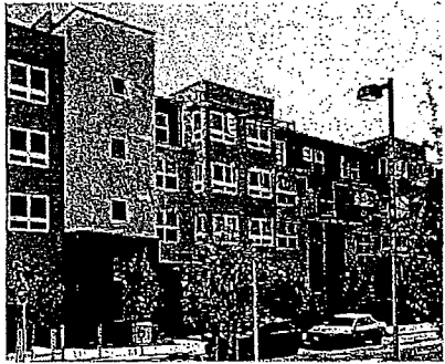
Exposed blank facades shall be architecturally treated to minimize impact.
