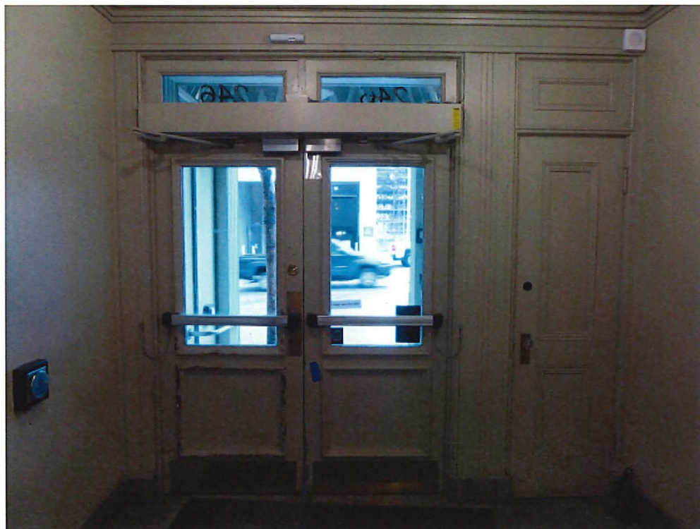
A17. View of vestibule and closet inside south entry, looking east (ARG, February 2017).
