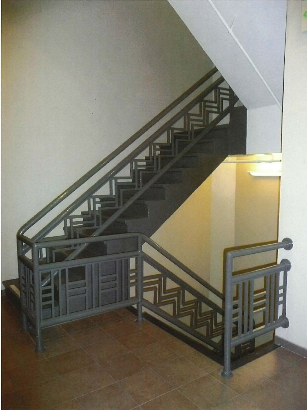
A20. View of metal stair with "zig-zag" pattern (ARG, October 2015).
