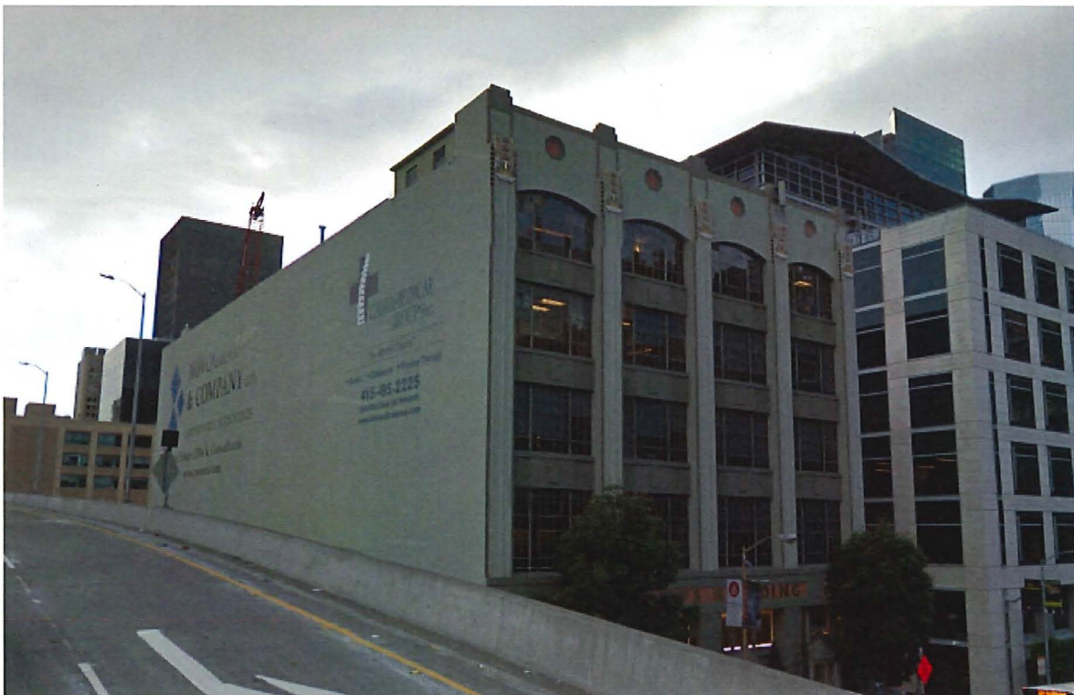
A10. View of south façade, looking west (Google street view, accessed October 2015).
