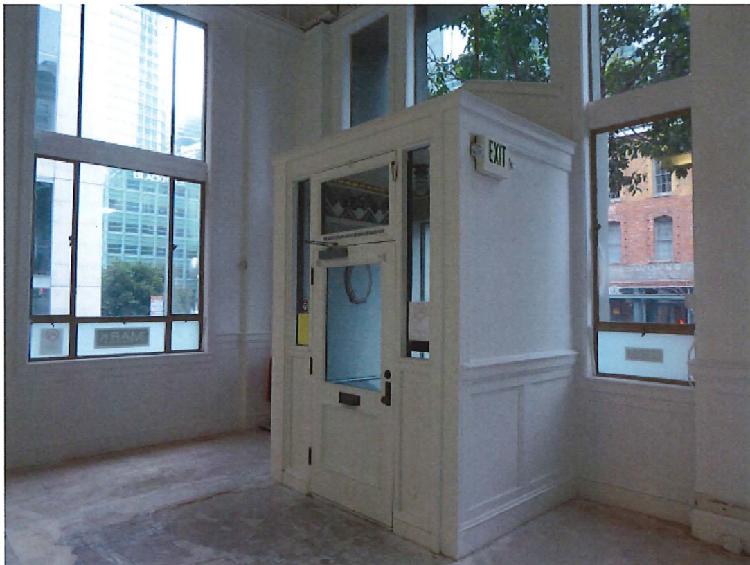
A13. Interior view of entrance at north end of front façade (ARG, February 2017). This area originally served as a display room and public space for the Phillips & Van Orden Company.
