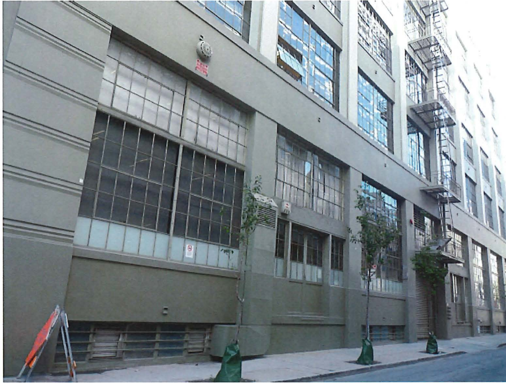
A5. View of north façade, looking south (ARG, October 2015).
