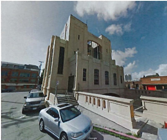
Posey Portal Superstructure, North End (Alameda and Oakland, 1928)
