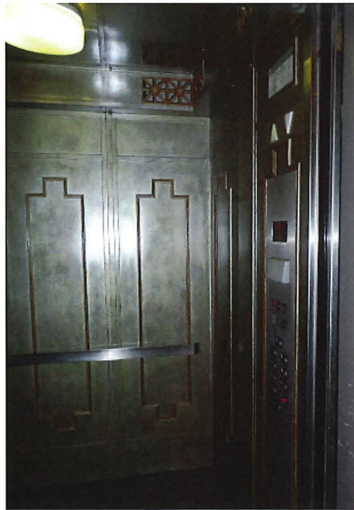
A19. View of interior of elevator cab (ARG, October 2015). Permit research and review of historic drawings did not confirm that the current metal panels are original.
