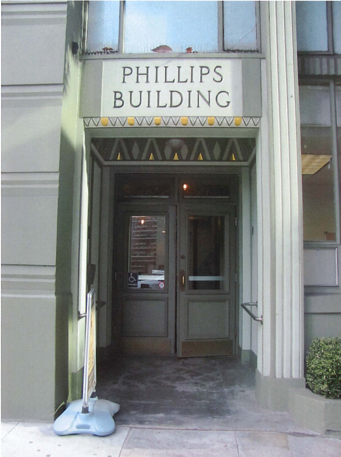
A11. Detail of entrance at south end of front façade (ARG, March 2016).
