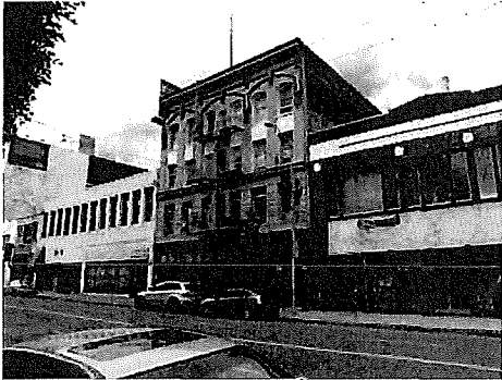
View of southeast and northeast facades.
