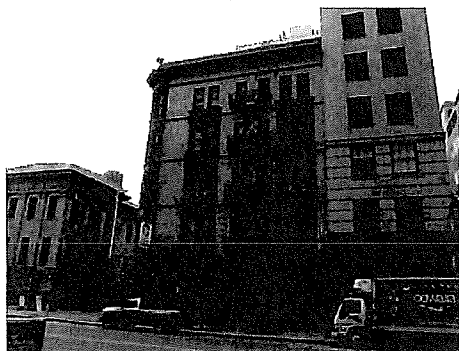
View of northeast facade. 103_4037.JPG 3/7/2011
