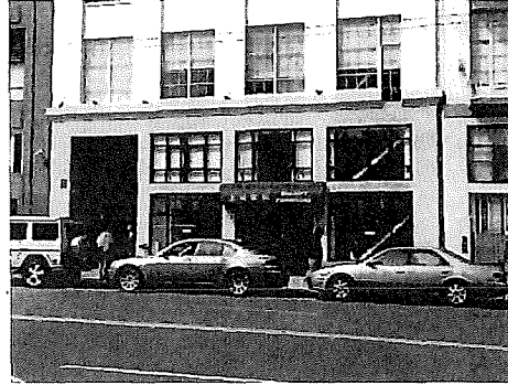
Detail of first story storefronts. 103_4083.JPG 3/8/2011
