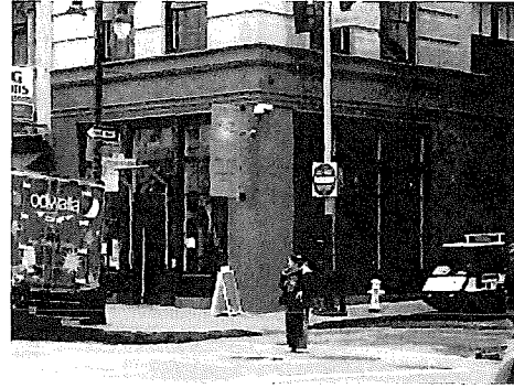
First story storefront. 103_4036.JPG. 3/8/2011
