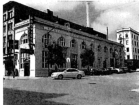
View of southeast and northeast facade. 103_4068.JPG 3/8/2011
