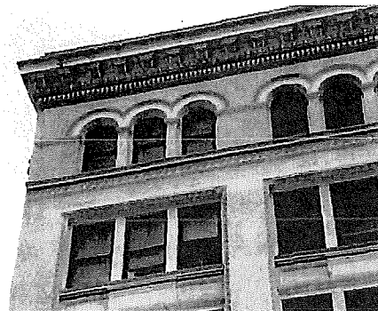
Detail of upper facade. 103_4096.JPG 3/8/2011
