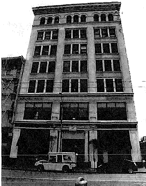
View of northwest facade. 103_4094.JPG, 3/8/2011
