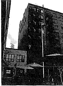
View of southwest and southeast facades. 103_4048.JPG 3/8/2011
