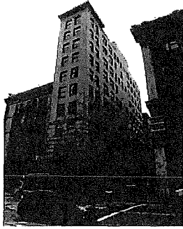
Fifth/Stevensen Street corner view, looking south. 103_4035.JPG. 3/8/2011
