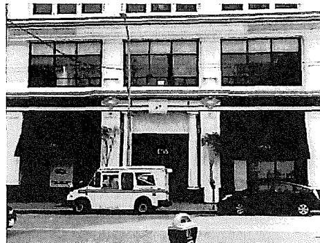
Detail of storefronts. 103_4095.JPG 3/8/2011
