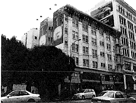
View of northeast and northwest facades.
