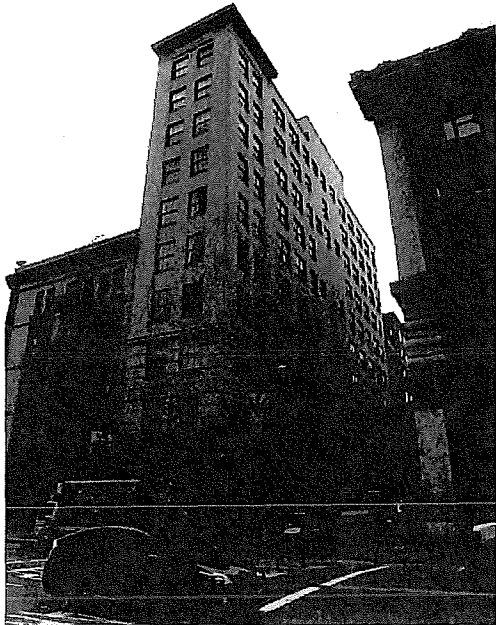
View of northeast and northwest facades. 103_4035.JPG 3/8/2011
