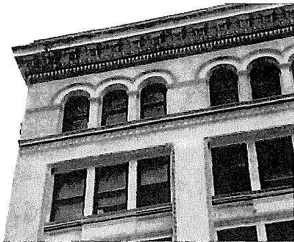
Detail of upper facade. 3/8/2011. 103_4096. JPG
