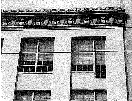
Detail of upper facade and cornice. 103_4082.JPG 3/8/2011
