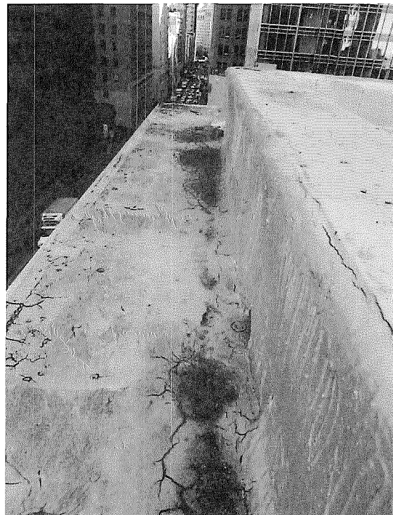
Figure 47: Detail view of parapet and top of cornice. Through-wall scuppers at the northern and eastern parapet walls drain the cornice back to the roof (photograph taken on 02/27/2018).
