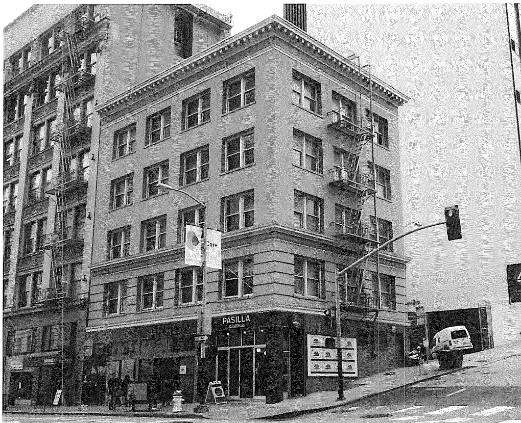
Figure 9: 353 Kearny Street viewed from intersection of Kearny and Pine Streets. Primary (east) facade and north facade (with fire escape) pictured. Looking southwest.
