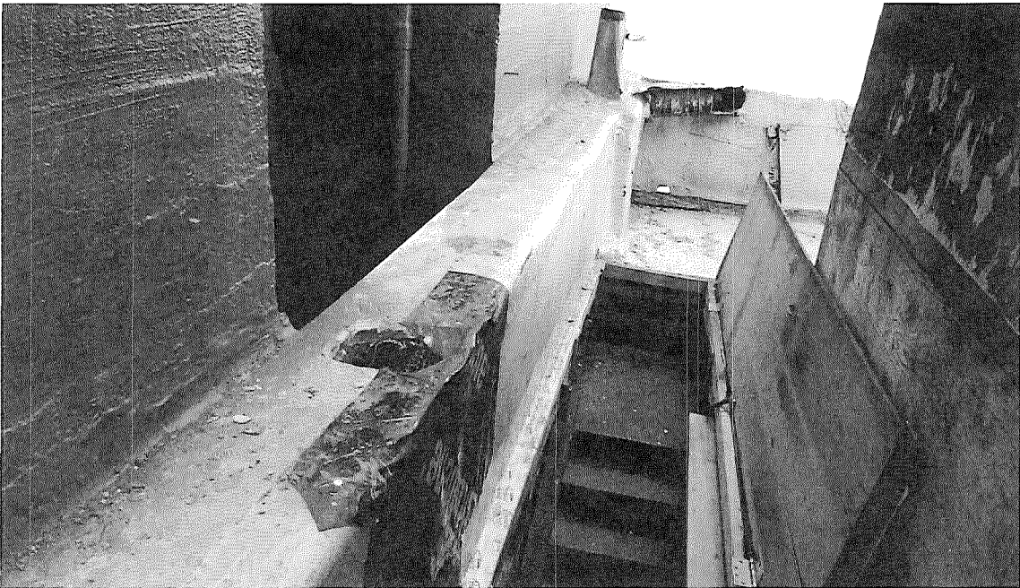
Figure 50: Photograph of roof access hatch located between elevator penthouse and southern parapet wall (photograph taken on 02/27/2018).
