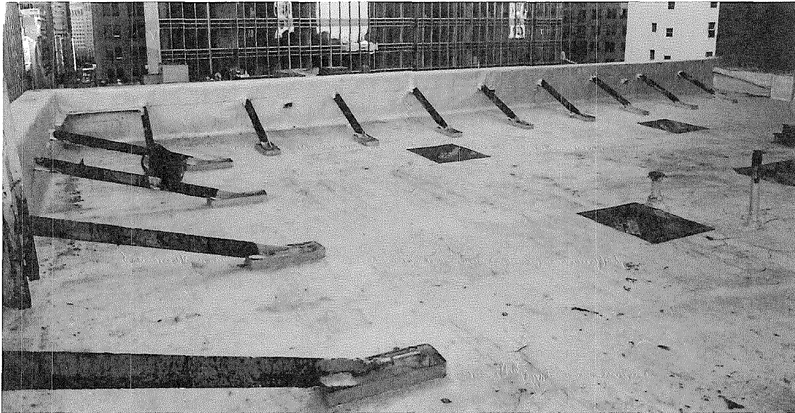
Figure 45: Photograph of built-up roof, looking east. Diagonal seismic bracing supports parapet walls (photograph taken on 02/27/2018).
