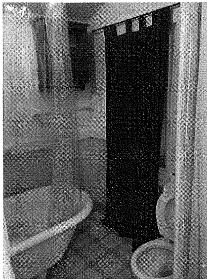
EXISTING BUILDING- BATHROOM
