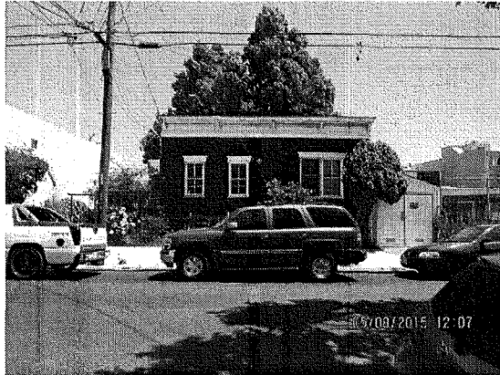
EXISTING BUILDING- LOOKING EAST
