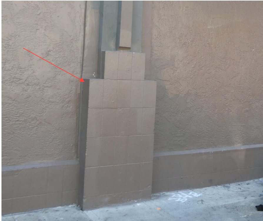
Figure 3: Chip no longer visible and has been painted over. (Page & Turnbull, 2024)
