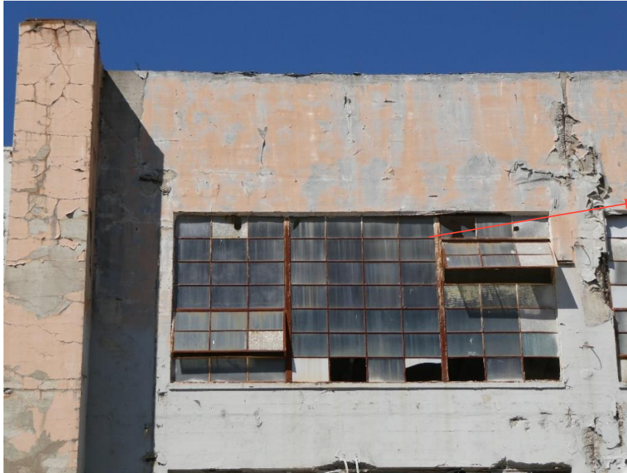
Figure 15: In the areas where the pipes were removed, the substrate was not properly patched and repaired, leading to cracks and spalls in the concrete and some exposed rebar. (Page & Turnbull, 2024)
