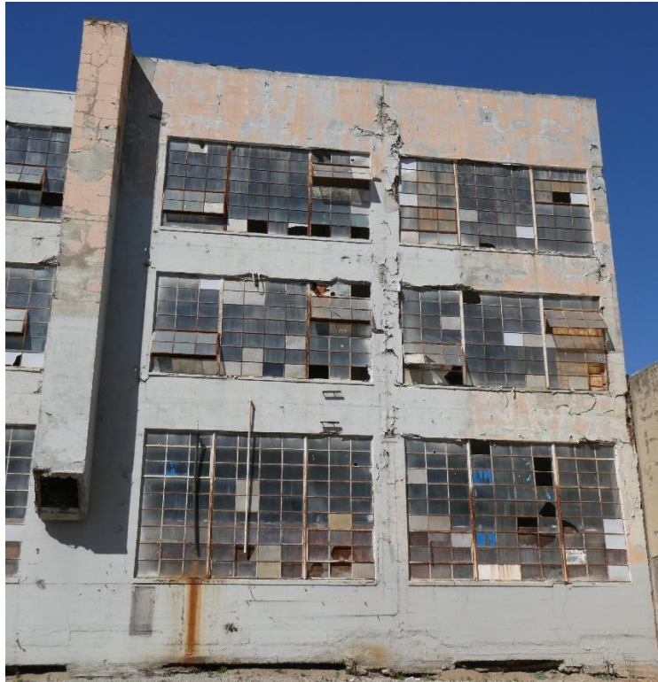
Figure 17: It appears that there are more broken, cracked, and missing window panes than is demonstrated in the 2018 report. (Page & Turnbull, 2024)
