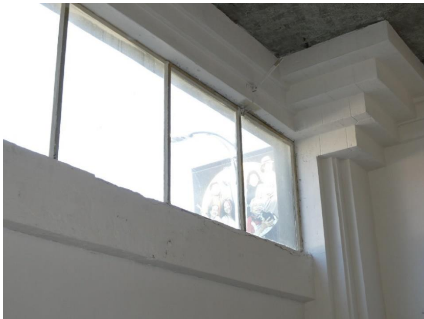
Figure 20: This leak and associated damage at the transom have been partially repaired and/or repainted. The area still exhibits damage and has areas of new paint failure. It is unclear if the source of the water intrusion has been fixed. (Page & Turnbull, 2024)
