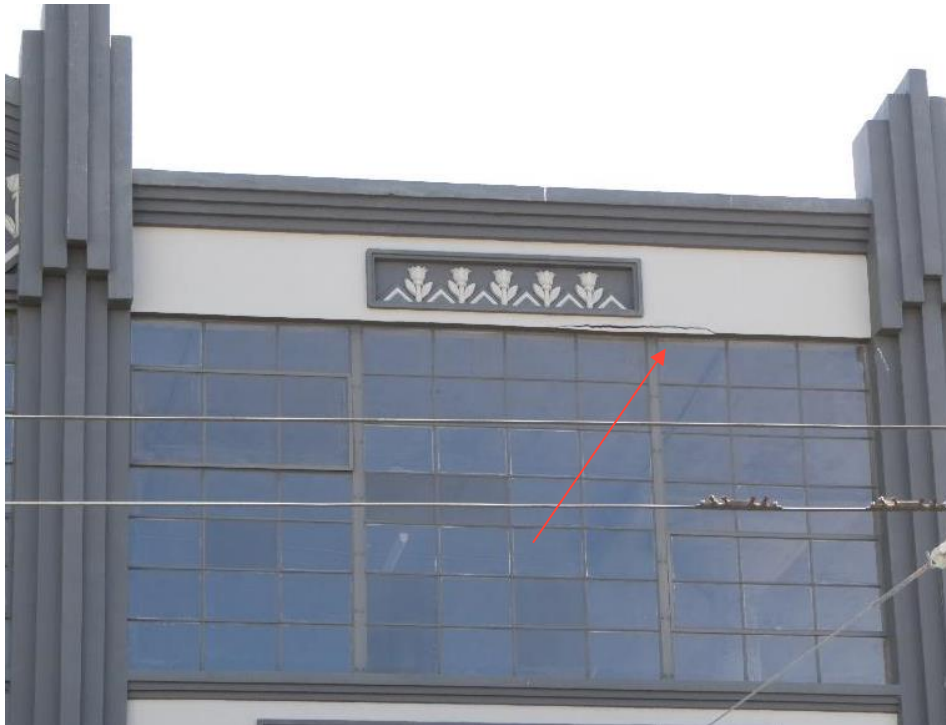
Figure 1: Incipient spall at the window head at the fourth bay from the east on the third floor. (Page & Turnbull, 2024)
