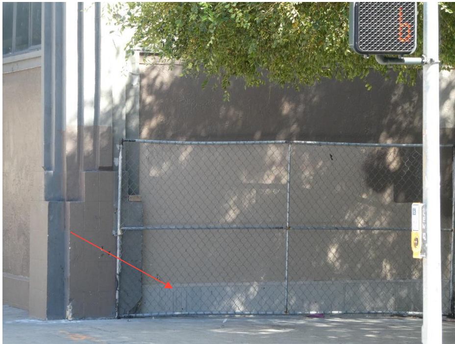
Figure 4: These tiles at the base have been removed from the west façade on the first and second bays from the north. These two areas have been infilled with concrete. (Page & Turnbull, 2024)
