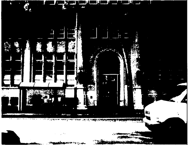
Otis Street Entryway
