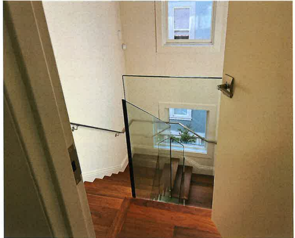
Enclosed secondary staircase (second means of egress)
