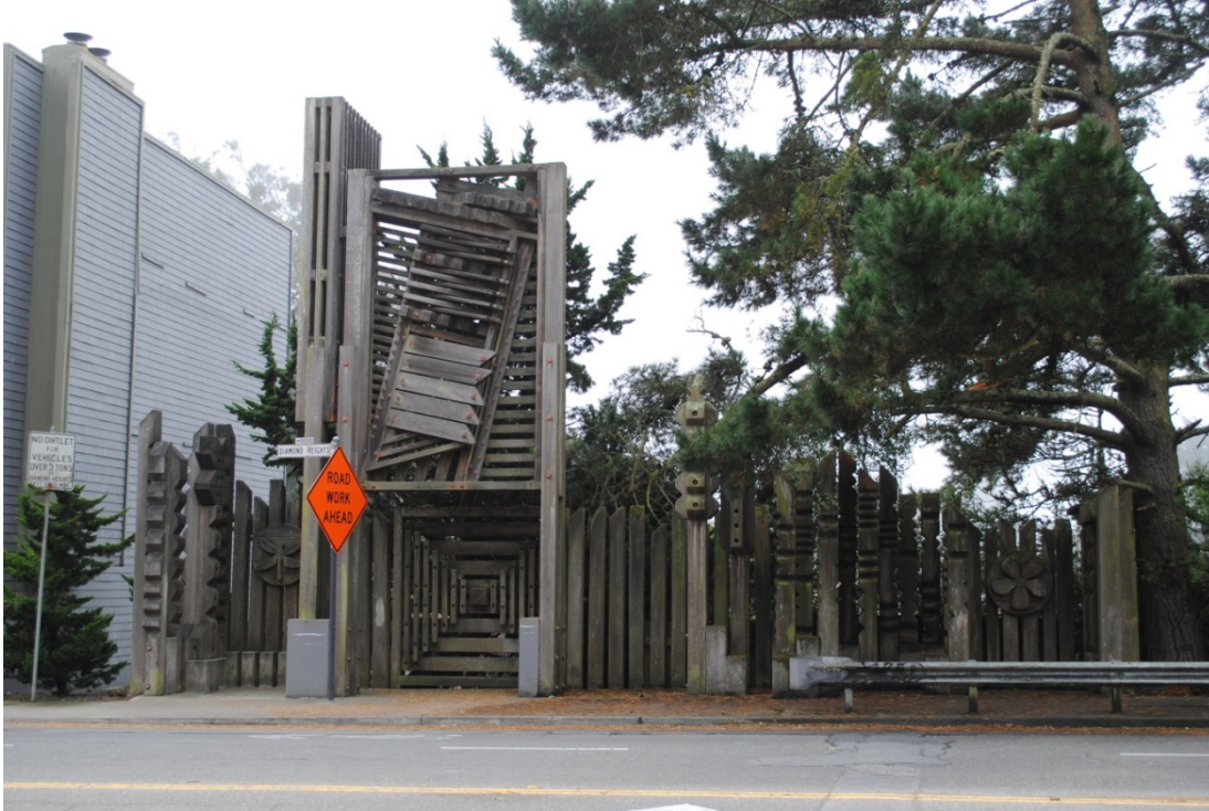
Primary (north) façade.
