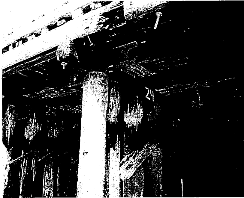
Photo 11--South Apron (repaired section)
