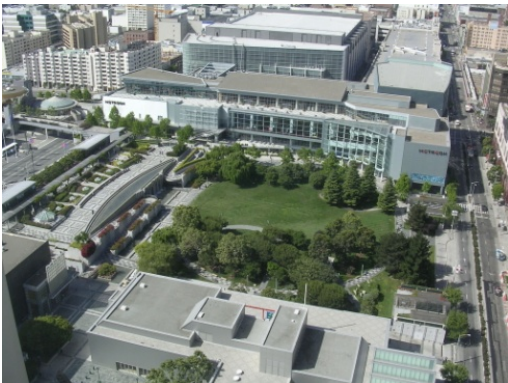
Aerial of Yerba Buena Gardens Open Space
