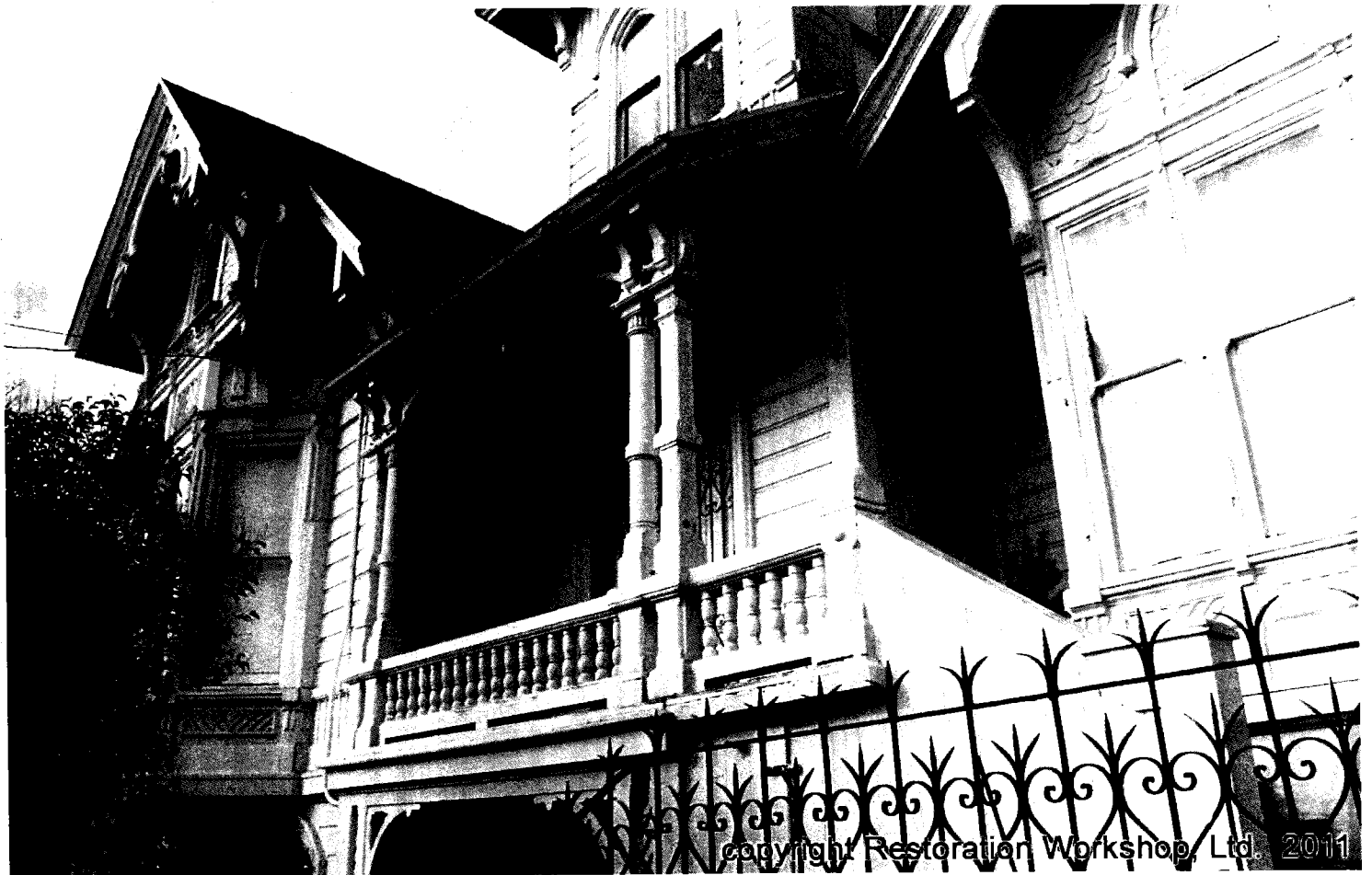
Eastern facade: Porch and main entrance.
