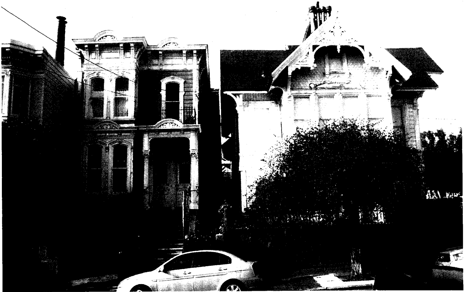
201 Buchanan ST: Waller Street (South) elevation and adjacent residence. Notice sheltered western facade
