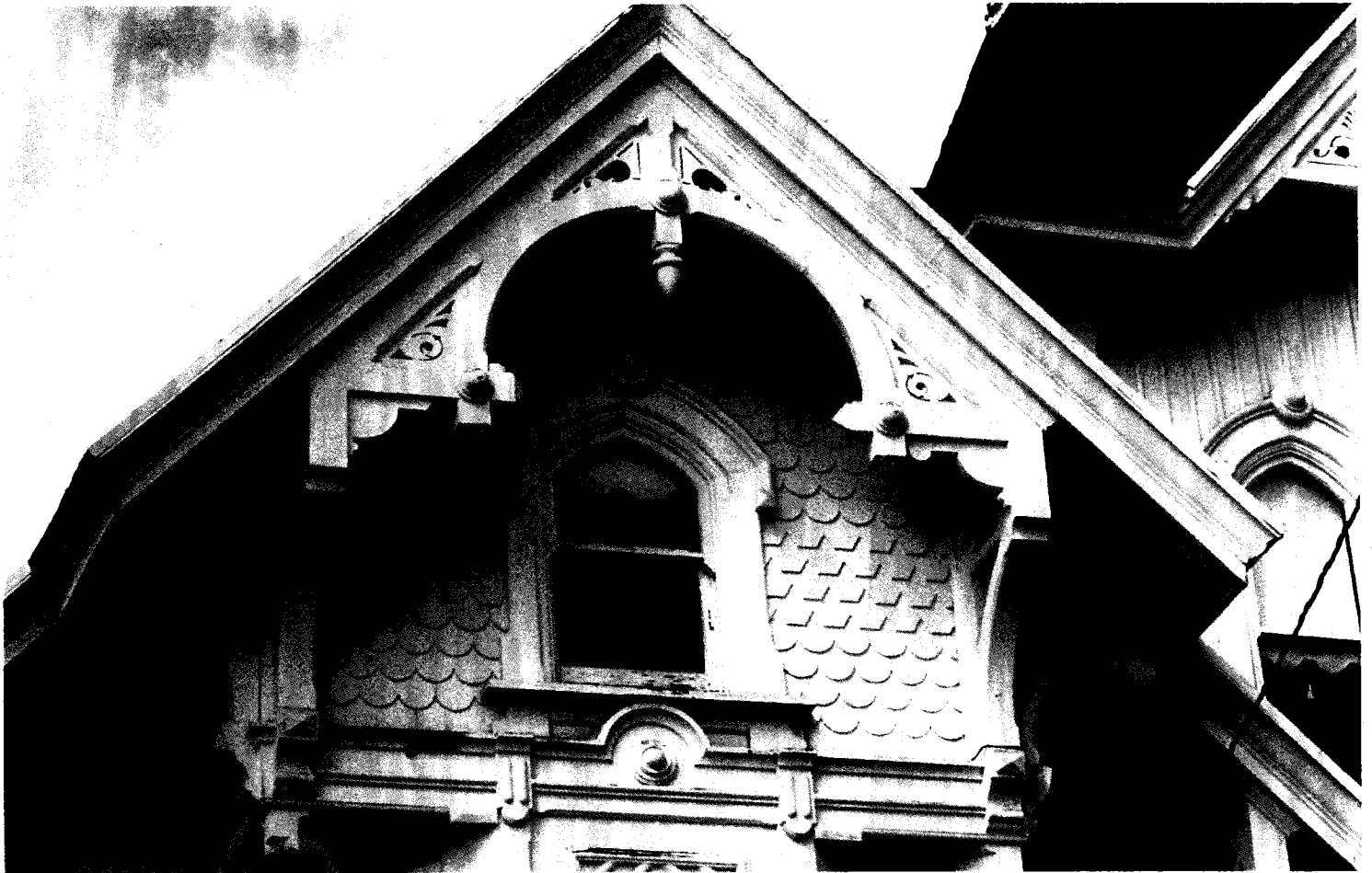
Gable over front parlor bay window (eastern facade).
