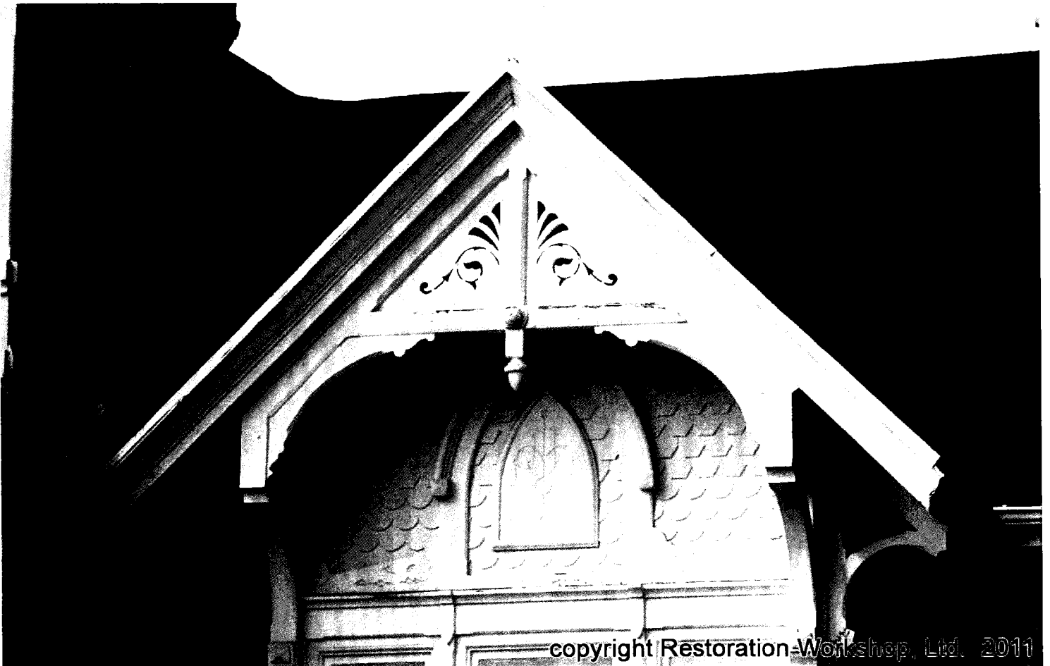
Gable over dining room bay (eastern facade)
