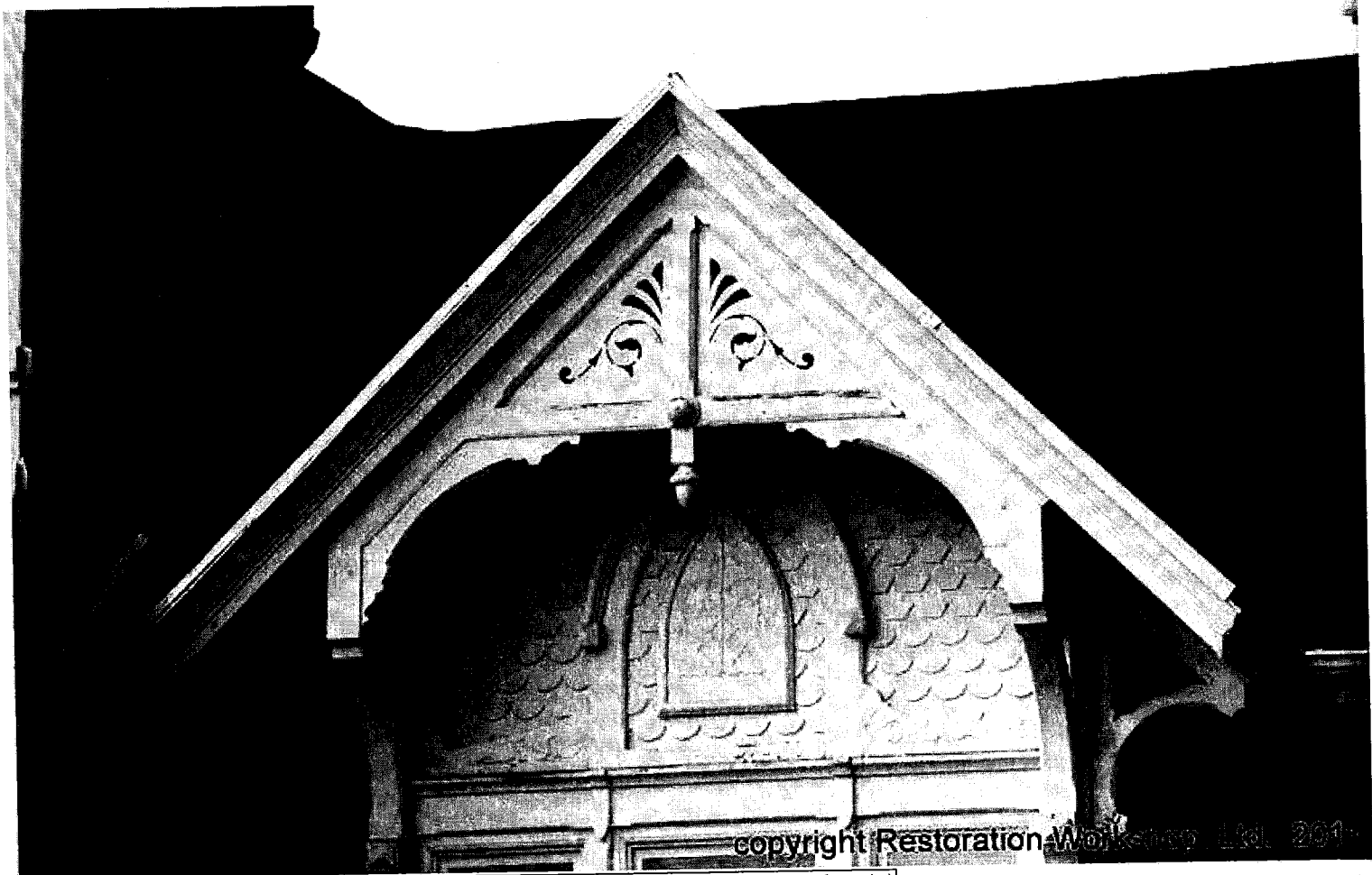
Gable over dining room bay (eastern facade)
