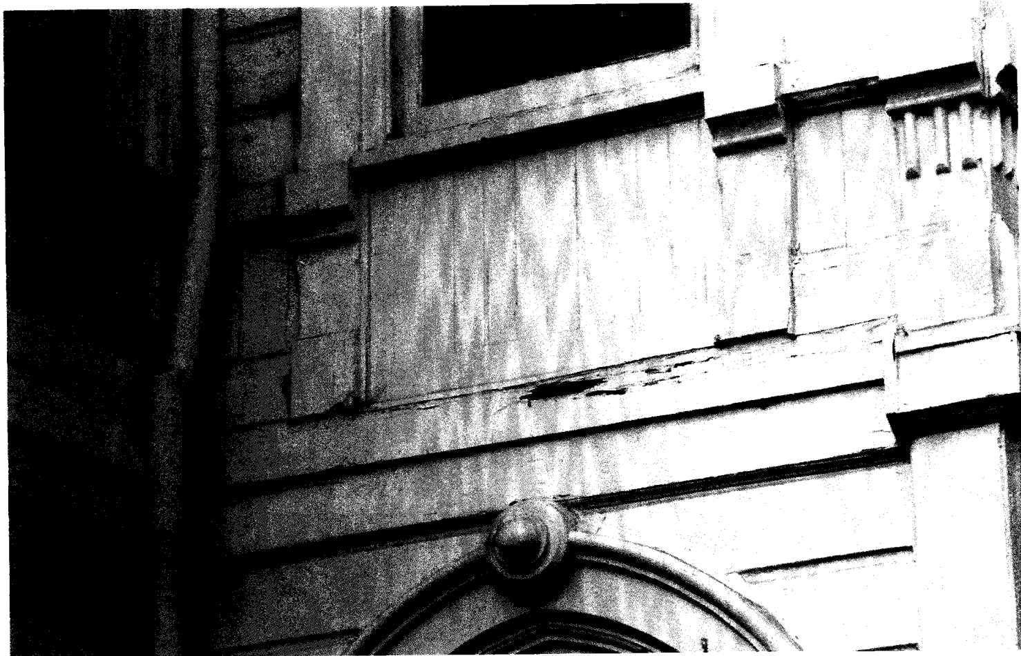
Former location of balcony east of sun room
