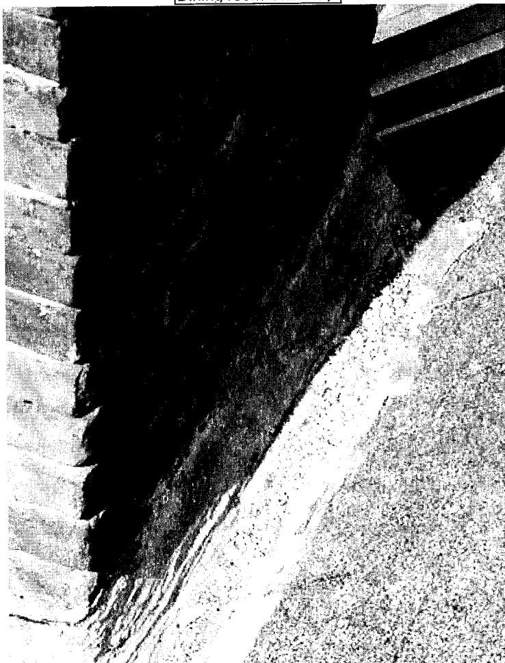
Base of Kitchen Chimney
