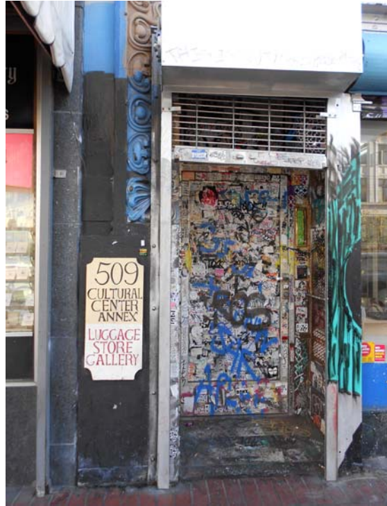
Figure 37. View southeast of door to main stairway. [No. 1323] January 2014.
