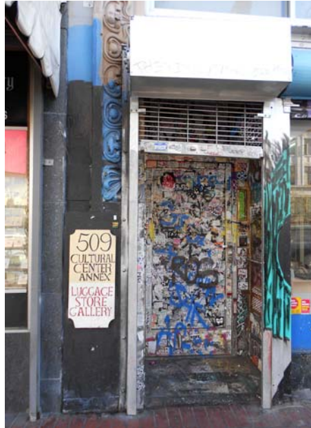
Figure 25. Doorway for 1007 Market Street. [No. 1323] January 2014
