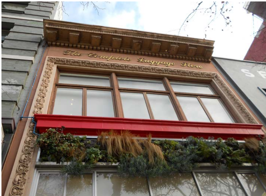
Figure 23. View of upper façade. [No. 15.56.41] January 2014.
