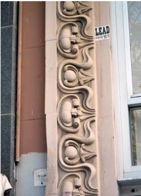
Figure 5. Detail of terra cotta molding around windows. [No. 15.56.15] January 2014.
