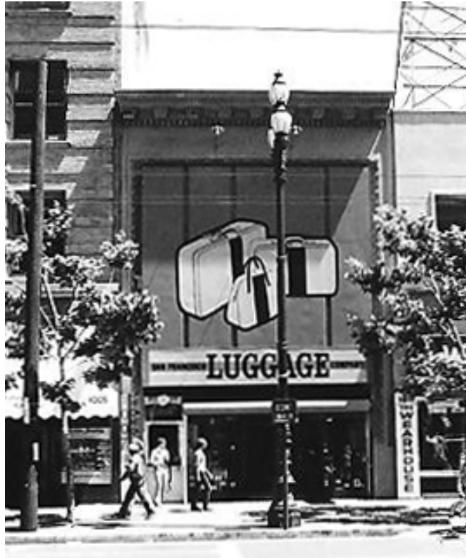
Figure 33. The Walker Building street façade with metal screen and sign over windows. Photo by Charles Hall Page & Associates, [No. 12.31.18] 1978.
