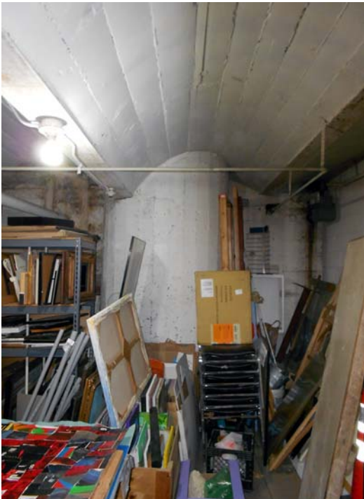
Figure 15. Interior view northwest in basement showing concrete sidewalk vault above and cylindrical manhole shaft under sidewalk. [No. 16.06.56] January 2014.
