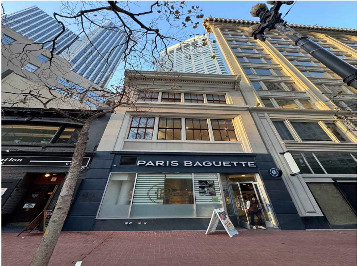
Subject block of Market Street (December 2024)
