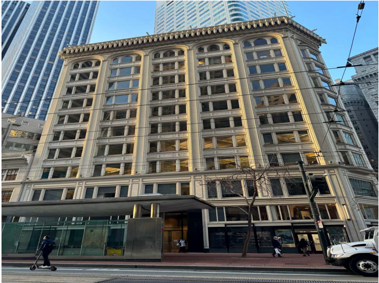
Subject block of Market Street (December 2024)
