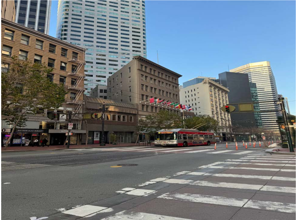
Subject property (570 Market Street) at center left (December 2024)
