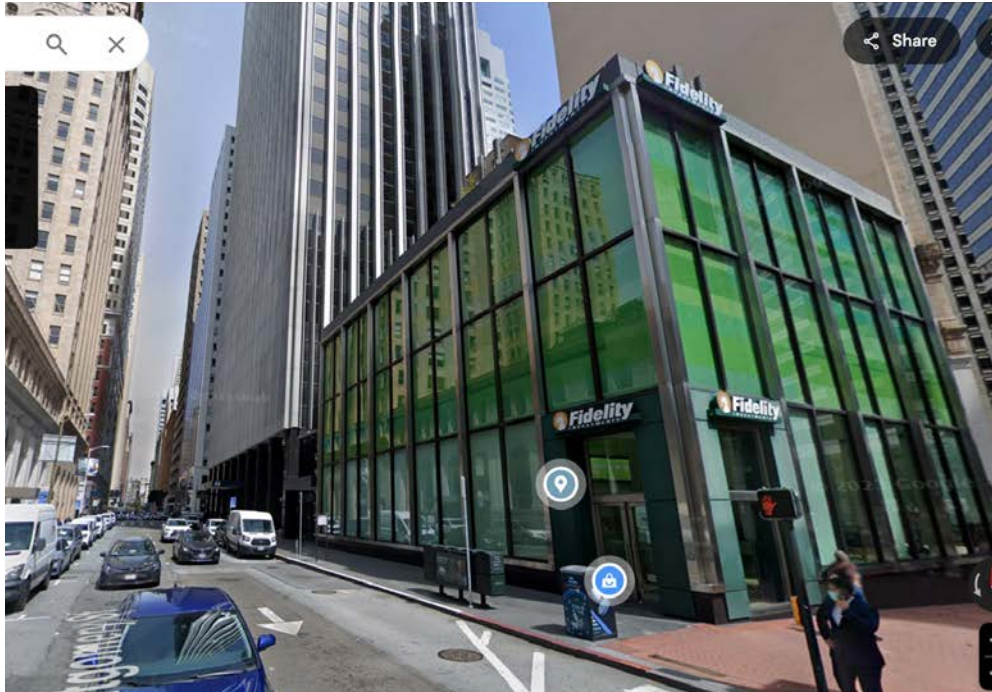
Montgomery Street side of subject block (2-44 Montgomery Street) (Source: Google, April 2023)
