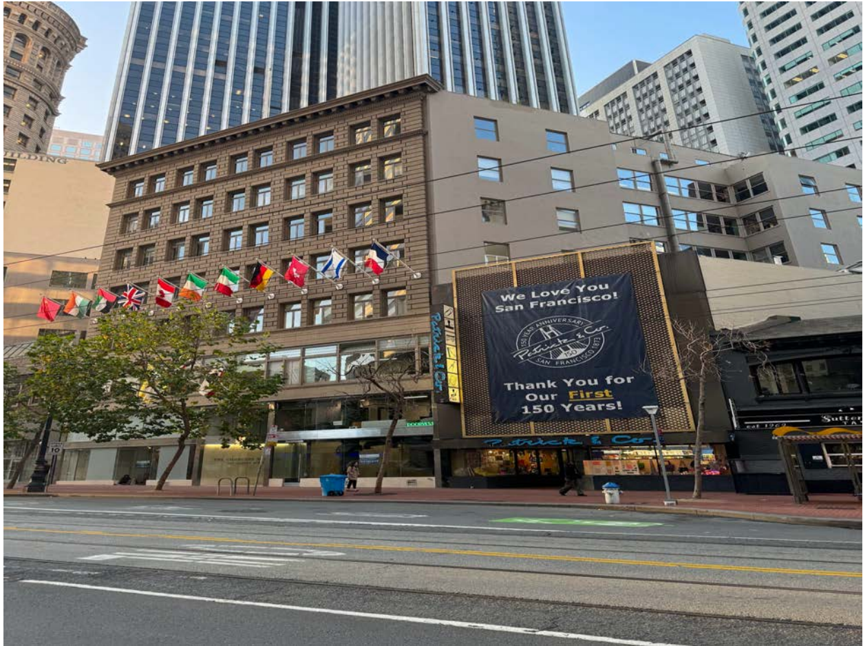
Subject block of Market Street (December 2024)
