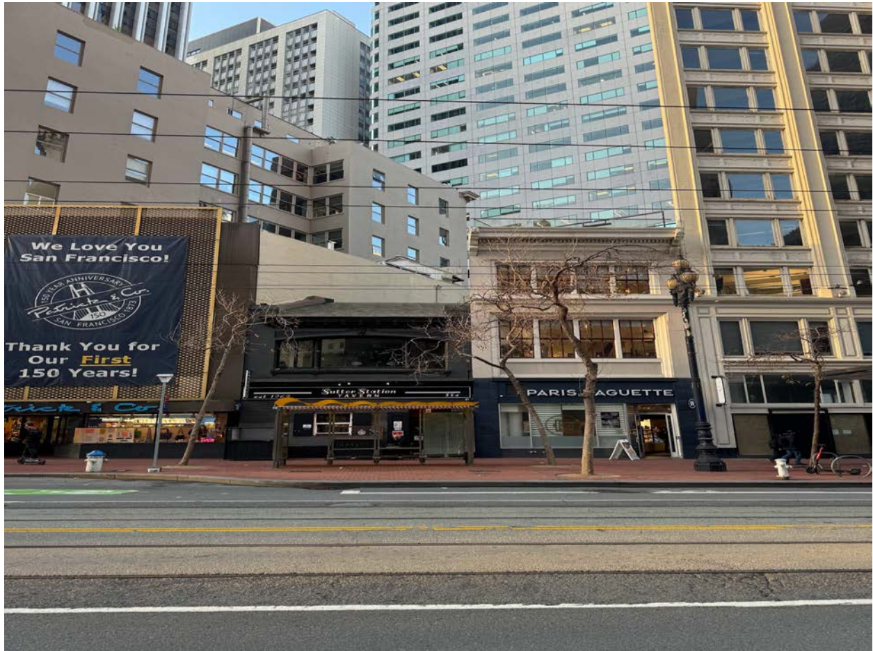
Subject block of Market Street (December 2024)
