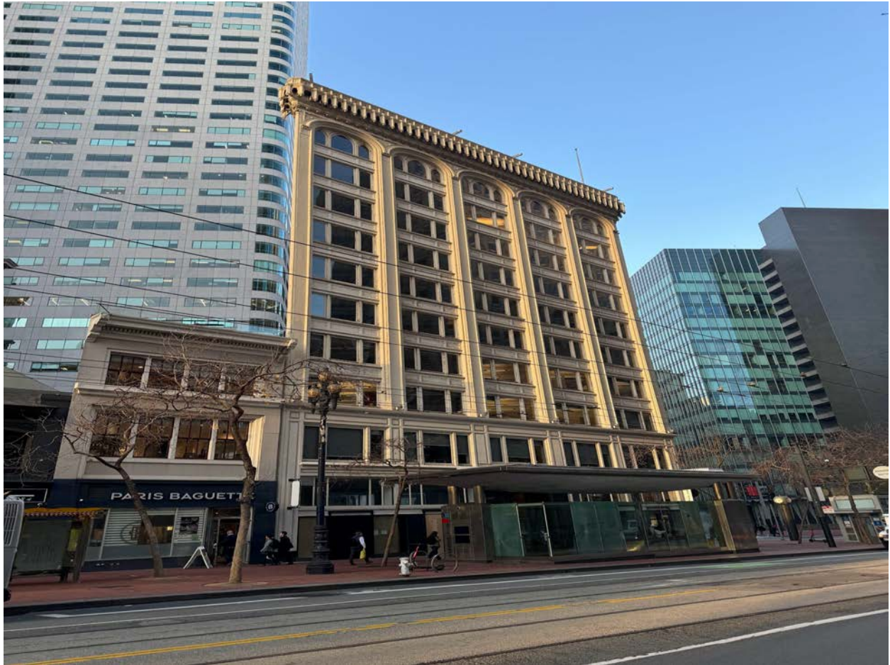
Subject block of Market Street (December 2024)
