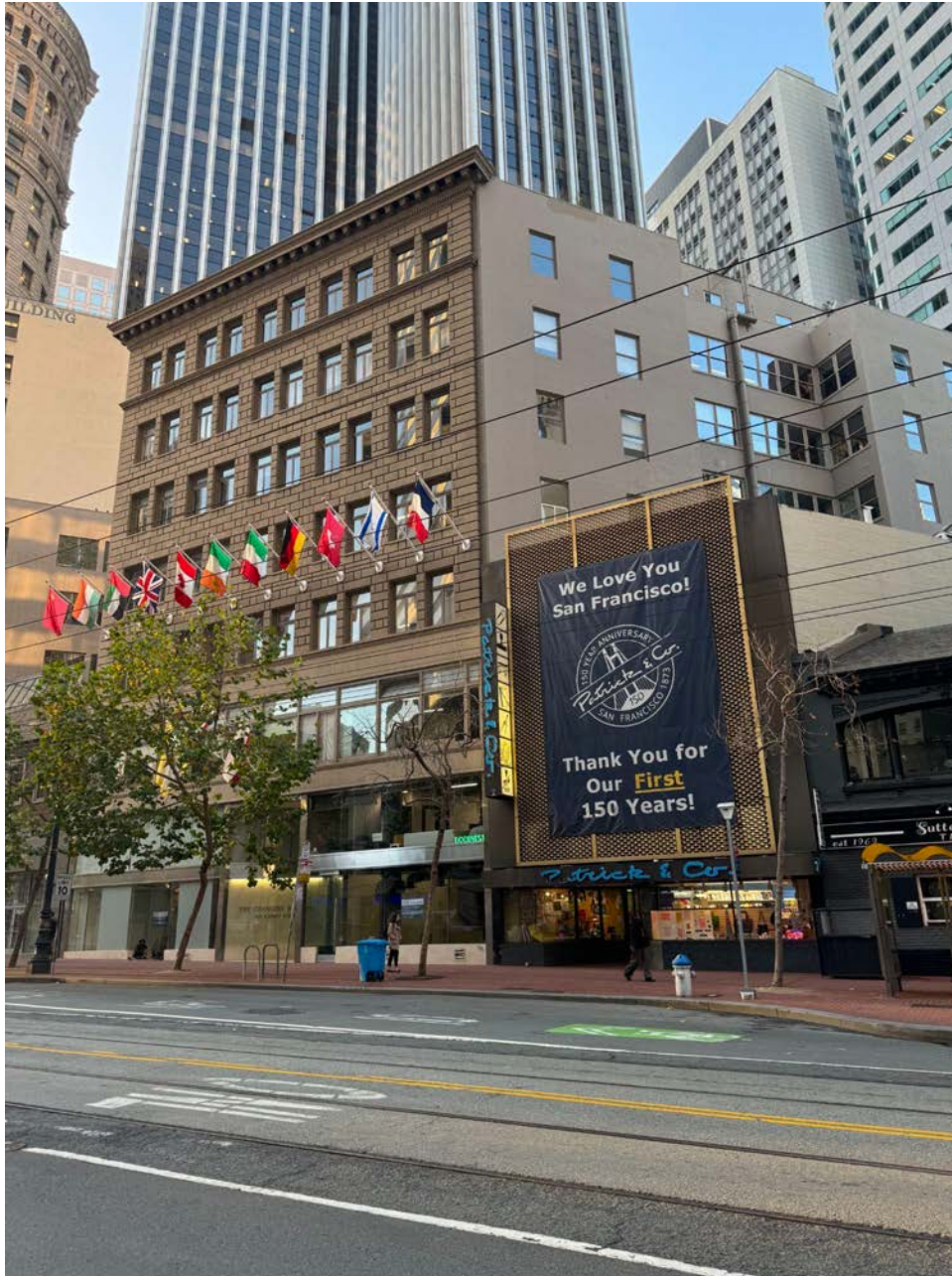
Subject block of Market Street (December 2024)
