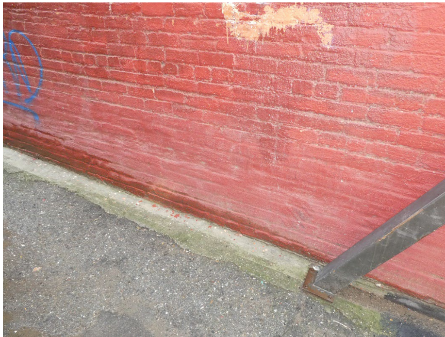
Figure 34: Parge coat and paint layer at the base of the masonry wall, west façade.
