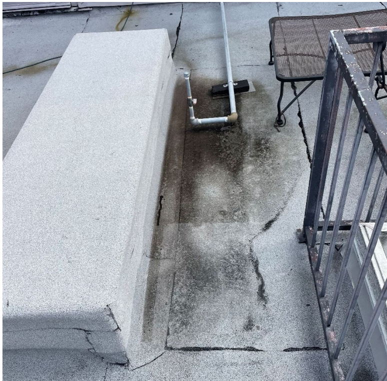
Figure 47: Active ponding on the main roof.
