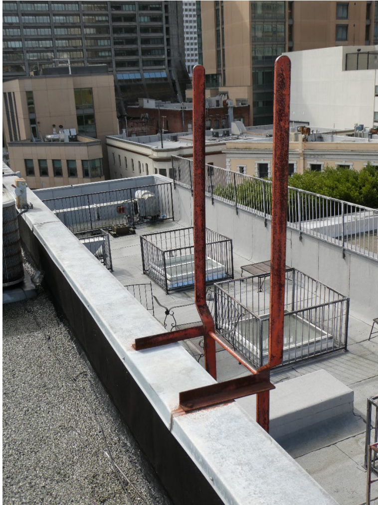
Figure 51: Rusted fasteners at the connection point between the ladder and parapet coping, penthouse roof.
