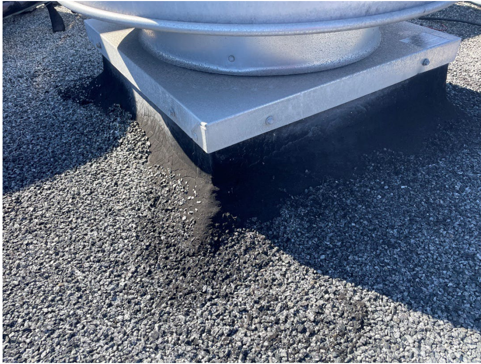
Figure 52: Alligatoring of the asphaltic roof coating, penthouse roof.
