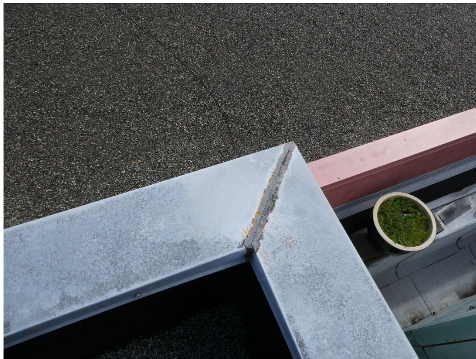
Figure 53: Deterioration of the joints at the roof coping, penthouse roof.
