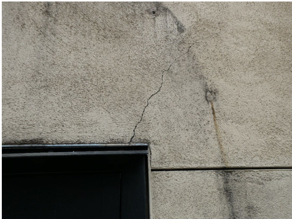
Figure 28: Diagonal crack originating from the corner of the door, south façade.
