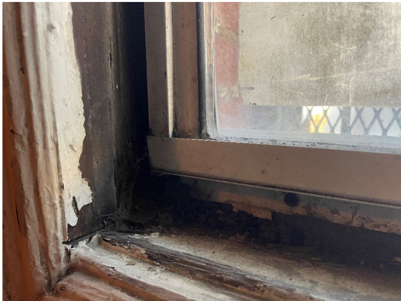
Image 34: View of wood frame deterioration at first floor, west wall. (Photo taken by P&T 03/14/2025)
