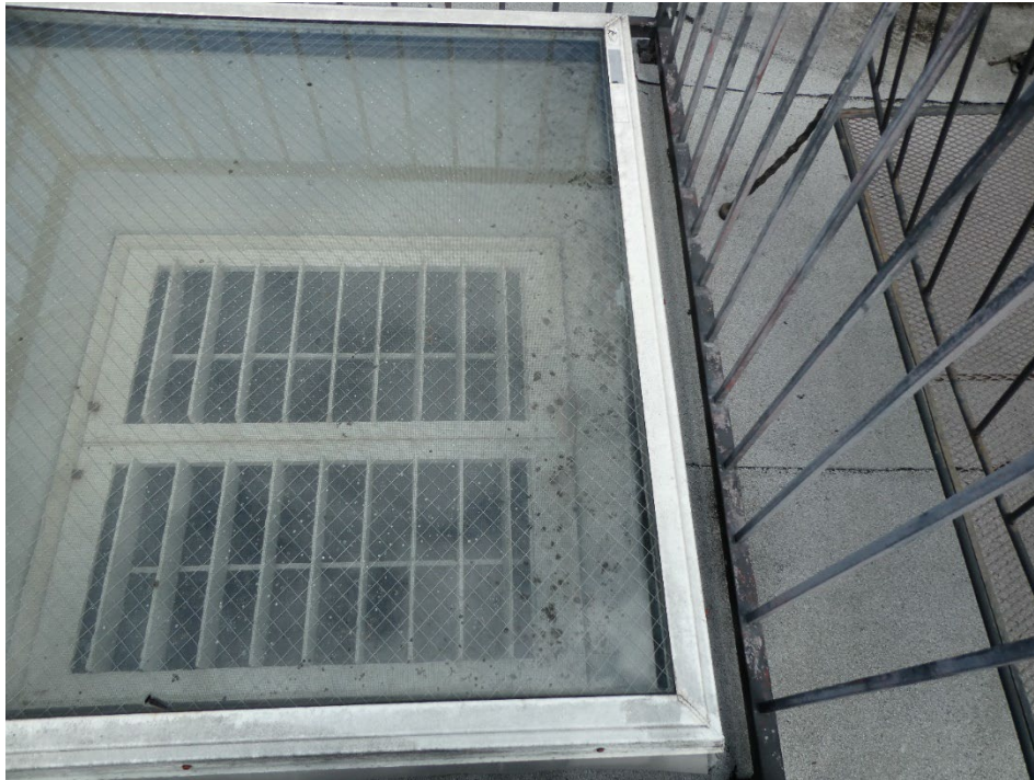
Figure 50: Ponding on top of the skylight and potential mold or mildew growth on the interior, main roof.
