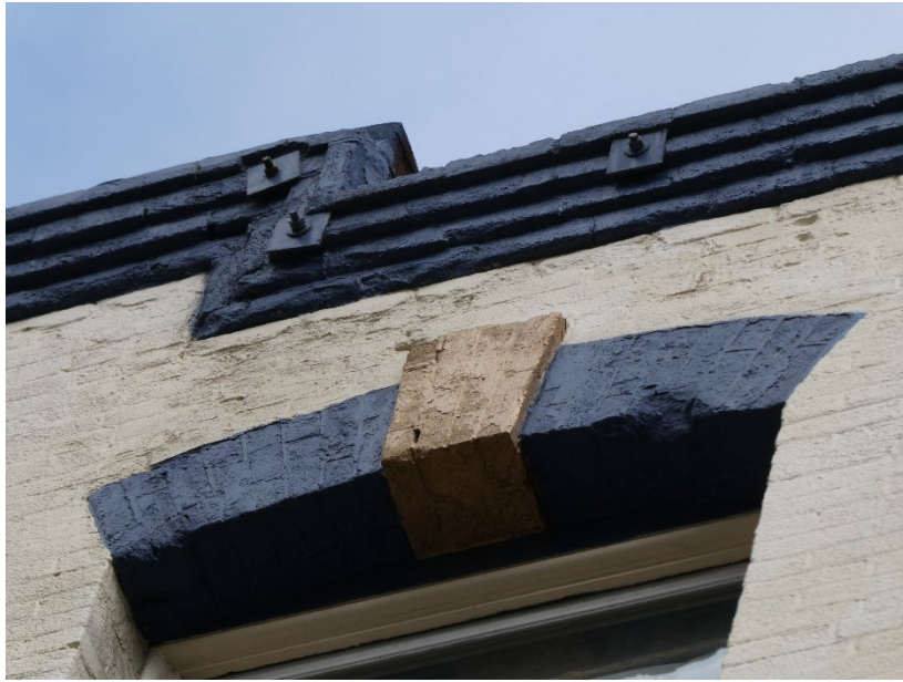
Image 11: Primary façade, painted masonry lintel and decorative parapet. (Photo taken by P&T 03/14/2025)
