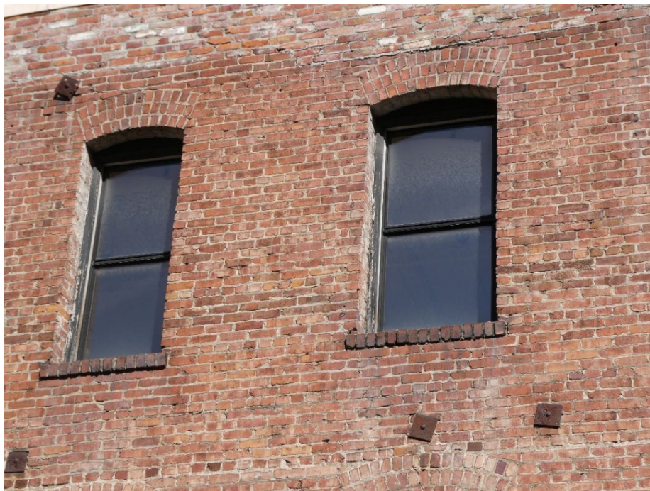
Figure 36: Third floor windows with historically incompatible aluminum frames and historic wood frames, west façade.
