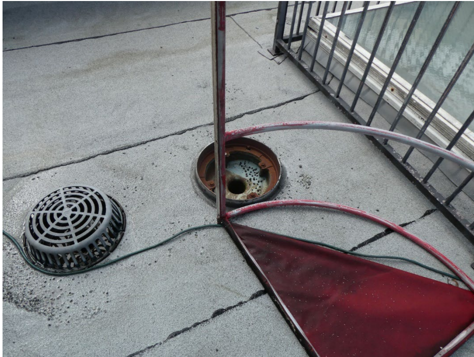
Figure 48: Missing drain cover, main roof.
