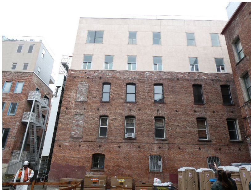
Image 4: View of 530 Jackson Street, west façade looking east. Historic masonry structure visible at floors one through three with stucco-clad metal stud structure at the fourth and fifth floors. (Photo taken by P&T 03/14/2025)
