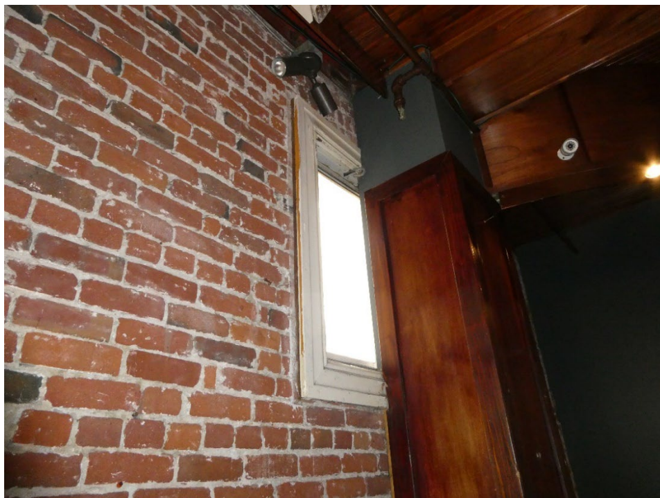
Figure 62: Historic window frame and trim with inserted non-historic window, first floor, west wall.
