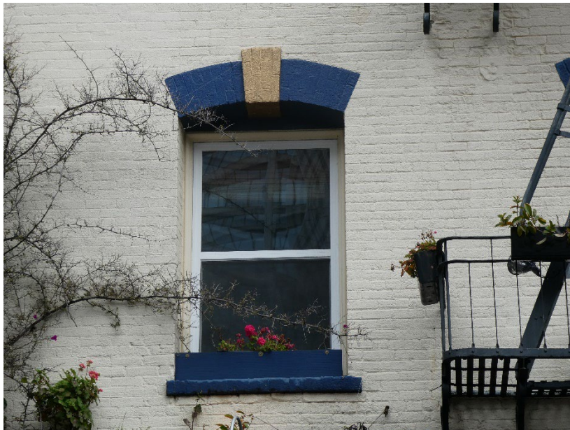
Image 12: Primary façade, typical vinyl replacement window in original masonry opening. (Photo taken by P&T 03/14/2025)
