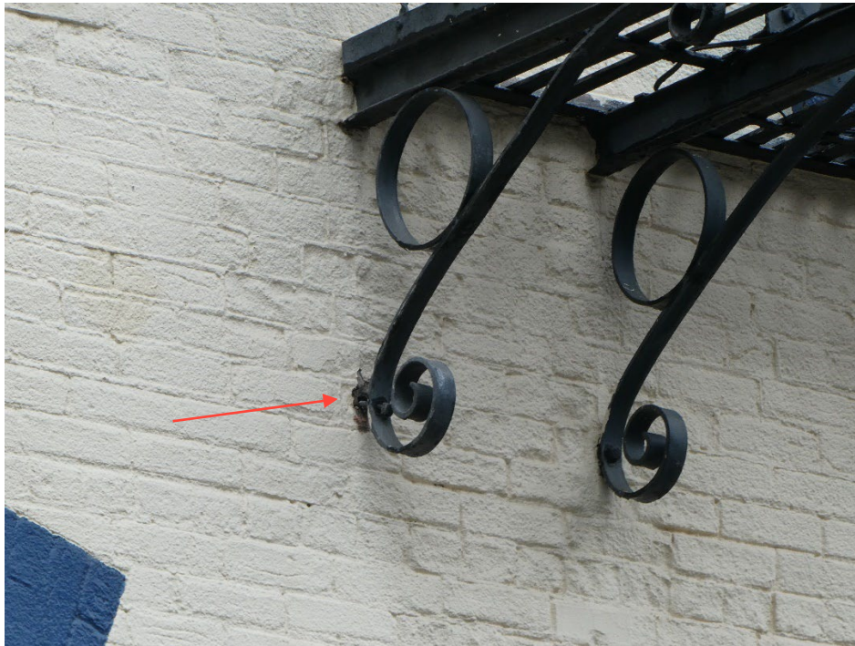
Figure 23: Loose anchor and masonry loss at the connection point between the masonry and the fire escape, above the second floor, south façade.
