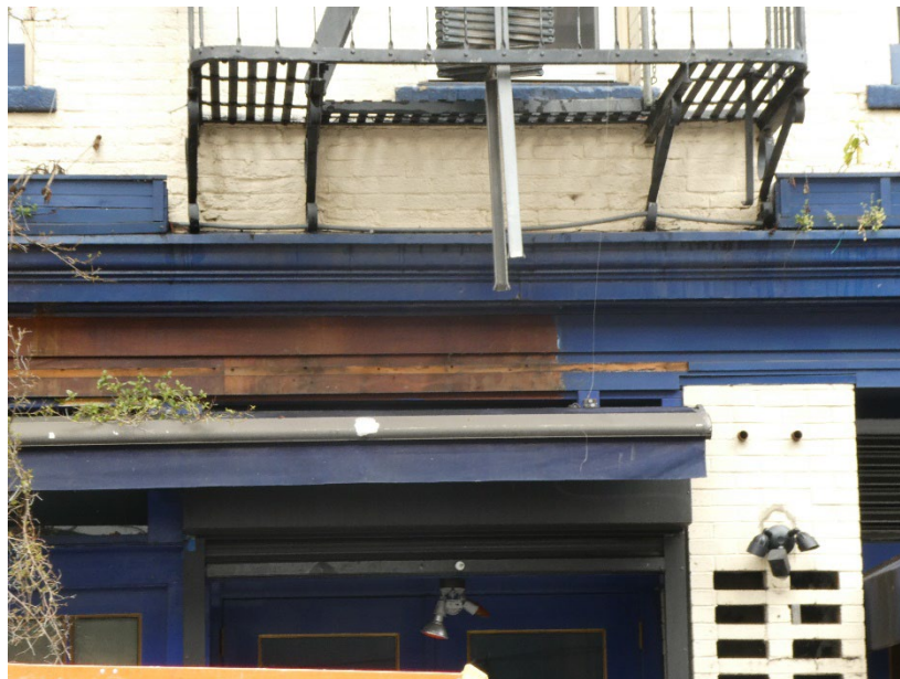
Image 10: Primary façade, wood and metal mid-band cornice above storefront. (Photo taken by P&T 03/14/2025)
