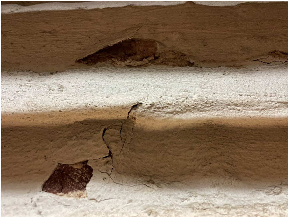
Figure 55: Paint loss at efflorescence, north wall, basement.
