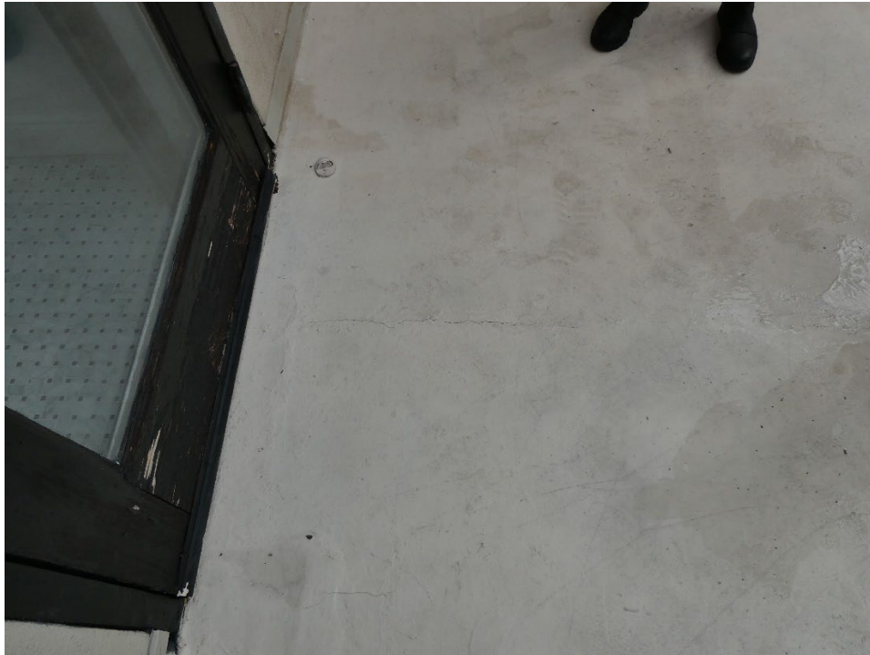
Figure 44: Cracking at the roof membrane, fifth floor balcony.
