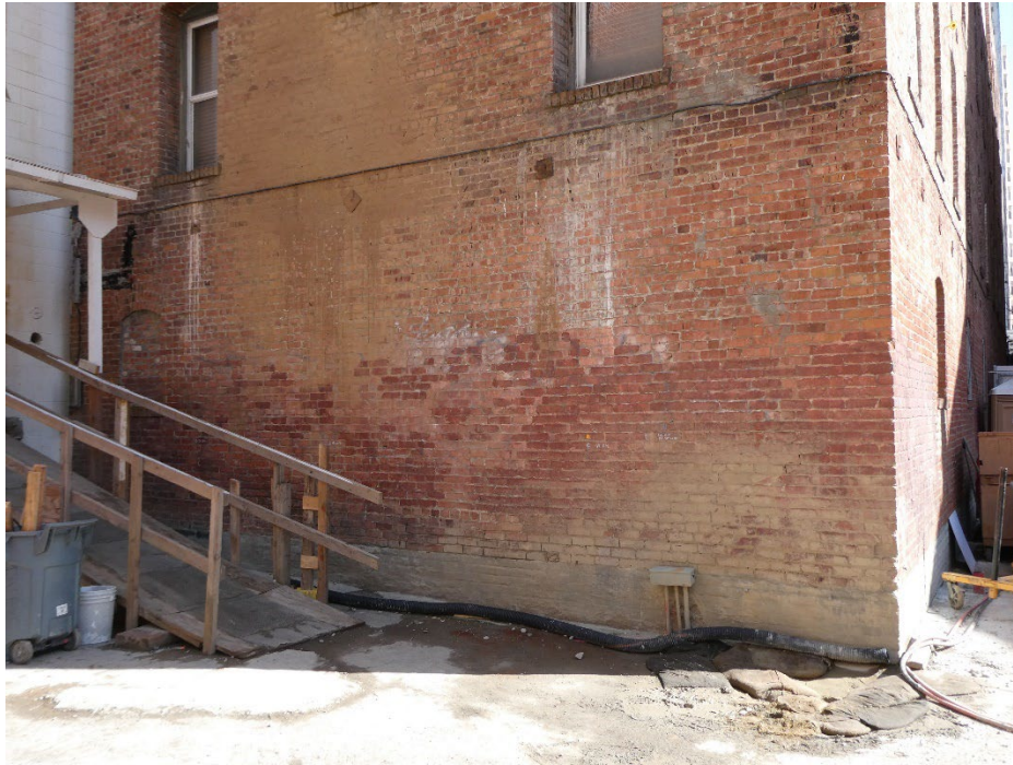
Figure 38: Water pooling at the base of the wall, mortar loss and extraneous paint and soiling on the masonry, north façade.
