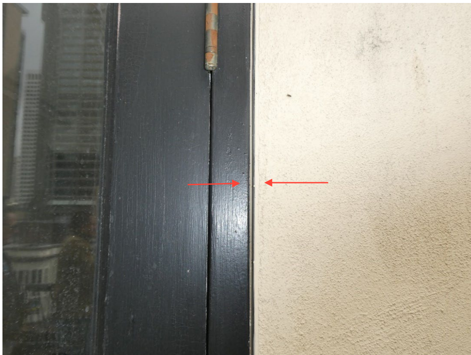
Figure 30: Open gap between the door frame and stucco, south façade.
