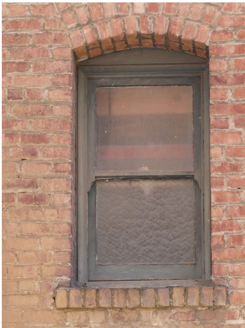
Figure 40: Original double-hung wood sash window at the second floor, north façade.
