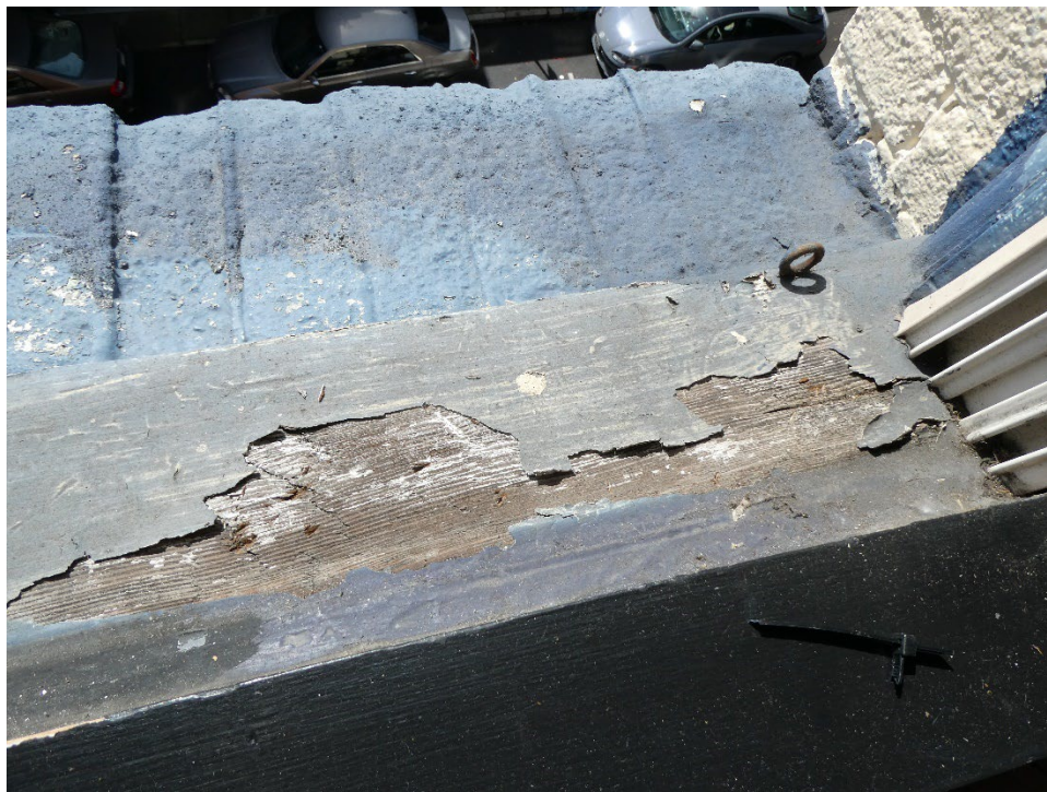
Figure 26: Paint loss exposing weathered wood with checking, UV damage, and raised grain at historic wood window sill, fourth floor, south façade.
