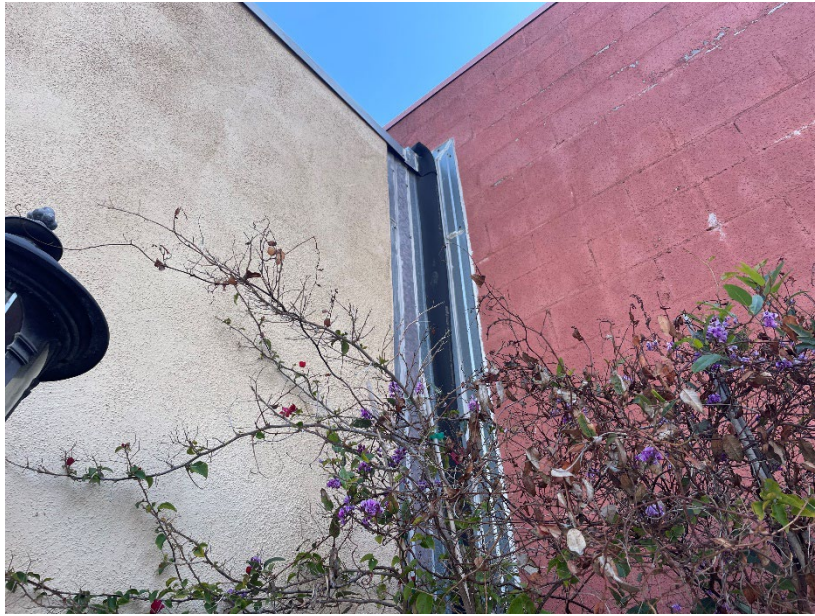
Image 19: Vertical seismic joint at east side of building, viewed from fifth floor balcony. Looking northeast. (Photo taken by P&T 03/14/2025)
