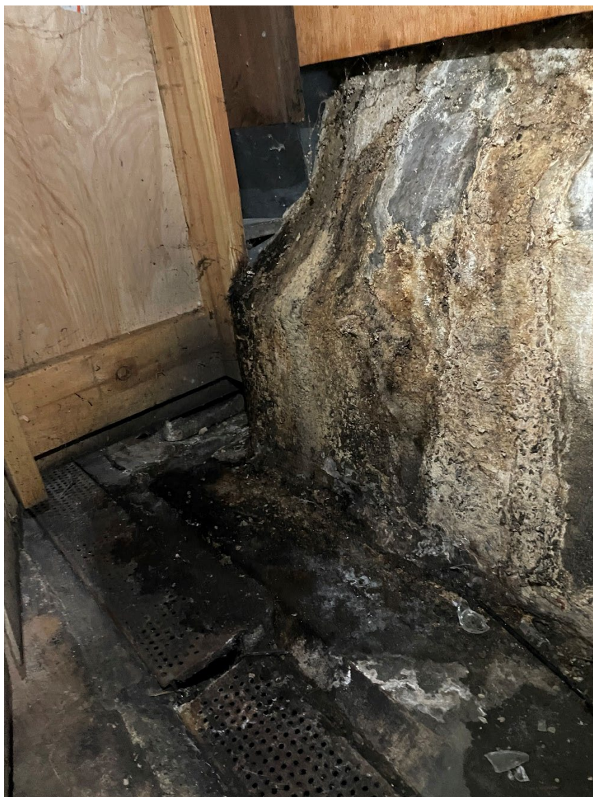
Figure 57: Active water infiltration and efflorescence, west wall, basement.
