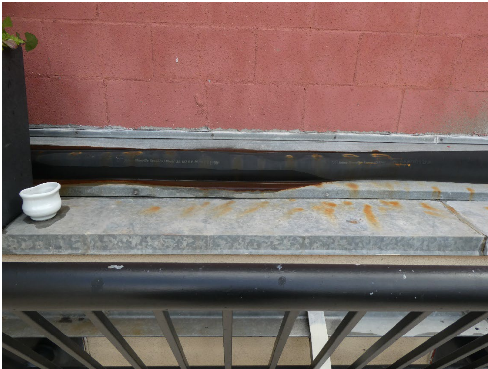
Figure 43: Surface corrosion at the metal coping/seismic expansion joint, fifth floor balcony.
