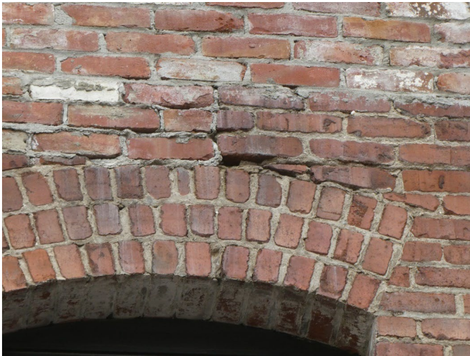
Figure 32: Mortar deterioration and loss at segmental arch, third floor, west façade.
