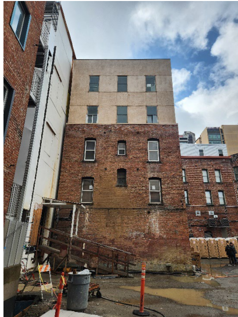
Image 3: View of 530 Jackson Street, north façade looking south. Historic masonry structure visible at floors one through three with stucco-clad metal stud structure at the fourth and fifth floors. (Photo taken by P&T 03/14/2025)
