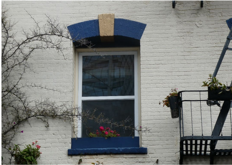
Figure 25: Second floor window with historically incompatible vinyl windows inserted into the historic wood frame, south façade.
