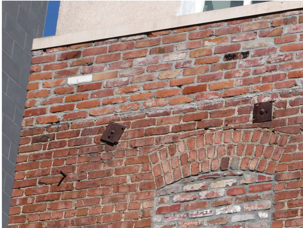
Figure 33: Tie rods with surface corrosion, west façade.
