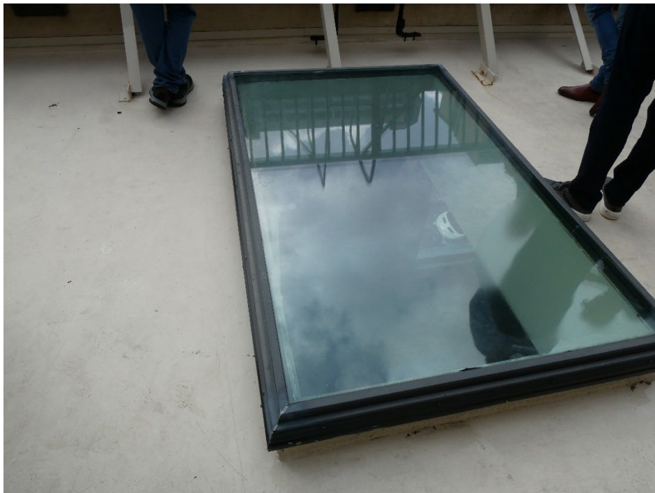
Figure 45: Skylight with no guard rail, fifth floor balcony.
