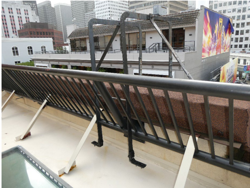
Image 17: View of fifth floor balcony, looking southwest. Diagonal parapet bracing and metal railing at forefront, fire escape ladder at center. (Photo taken by P&T 03/14/2025)
