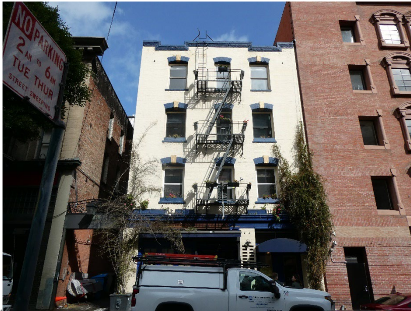
Image 1: Overall view of 530 Jackson Street primary façade. Wood and glass storefront system on first floor with masonry façade and double hung windows in openings on floors two through four. (Photo taken by P&T 03/14/2025)
