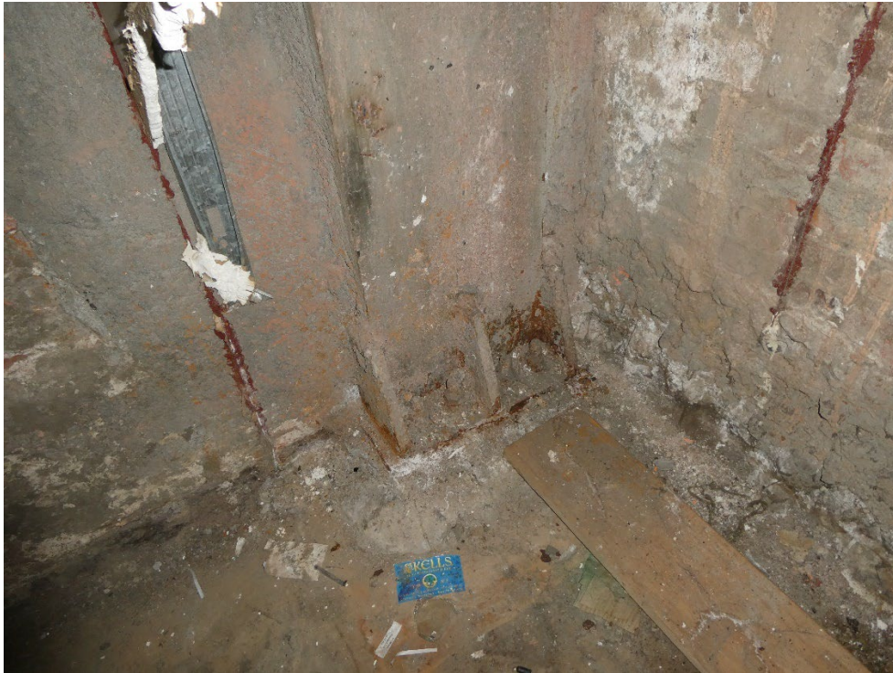
Figure 60: Corroded iron column base, basement.
