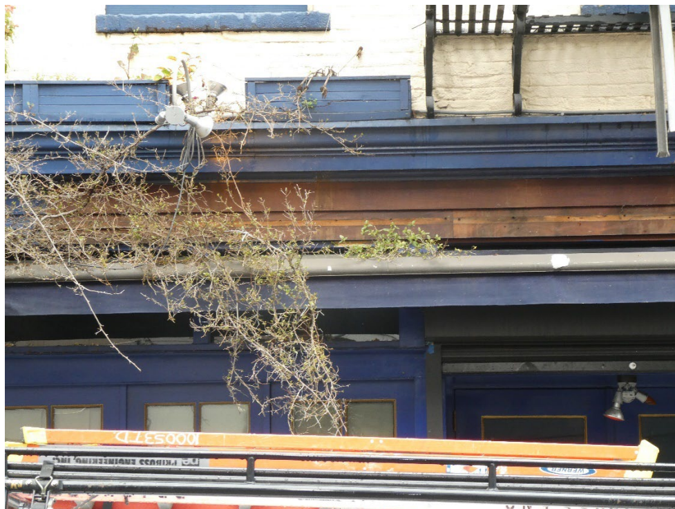
Figure 22: Unpainted area of wood at the mid-band cornice, south façade.
