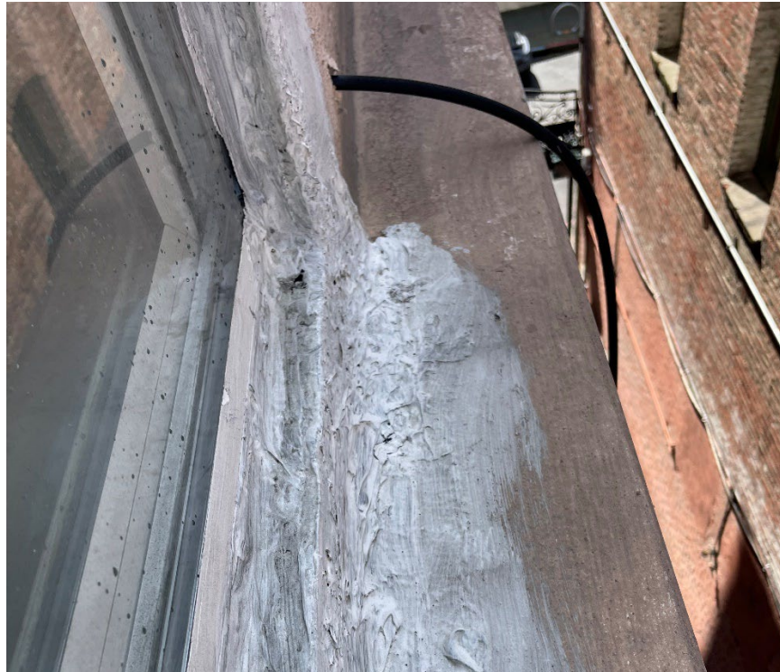
Figure 35: Deteriorated metal coping and large build-up of sealant around windows, fourth floor, west façade.
