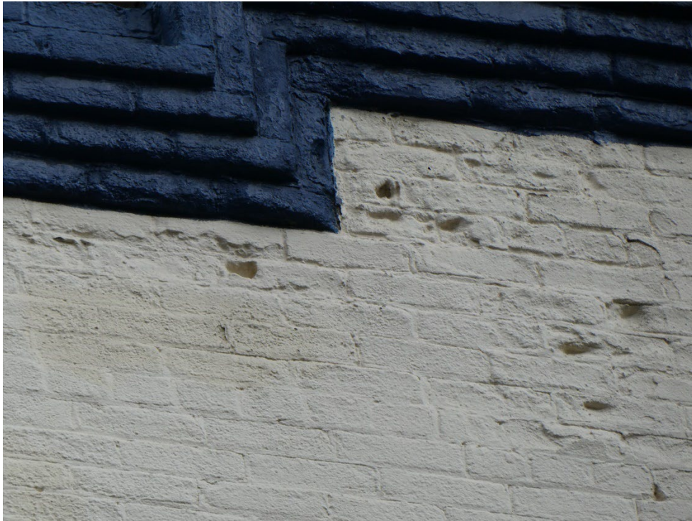
Figure 21: Brick and mortar deterioration at the parapet, Jackson Street (south) façade.
