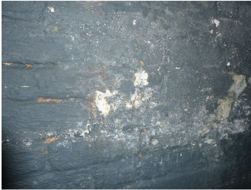
Figure 56: Efflorescence and paint loss on masonry west wall, basement.
