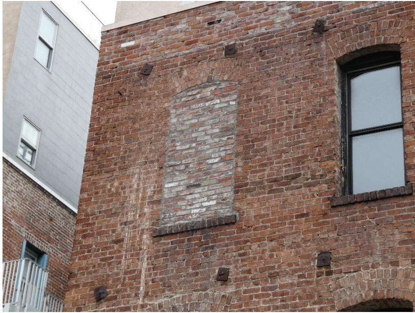
Image 13: Northwest exterior corner, looking east. Typical brick infill at historic masonry opening, third floor. (Photo taken by P&T 03/14/2025)
