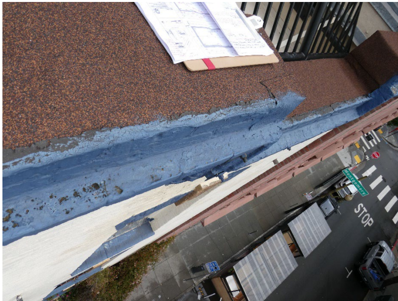
Image 18: Asphaltic roof flashing at masonry parapet, fifth floor balcony, looking down, east. (Photo taken by P&T 03/14/2025)
