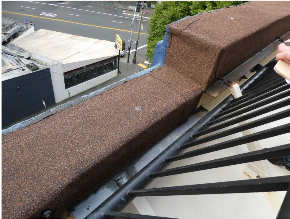
Figure 42: Some deterioration of the seams at the asphaltic coping at the south parapet wall, fifth floor balcony.
