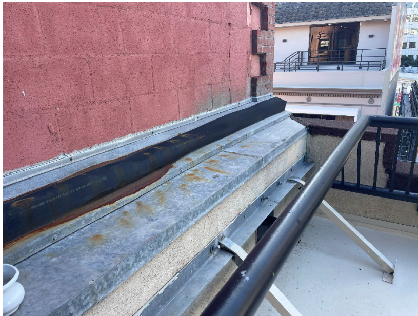
Image 20: Horizontal seismic joint at east side of building, viewed from fifth floor balcony. Looking south. (Photo taken by P&T 03/14/2025)
