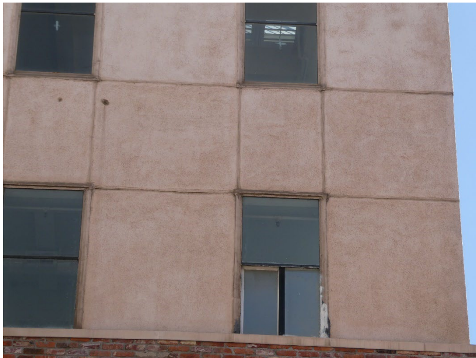
Figure 39: Deteriorated and poorly installed windows at the fourth and fifth floors, north façade. Note failed joints at the stucco.
