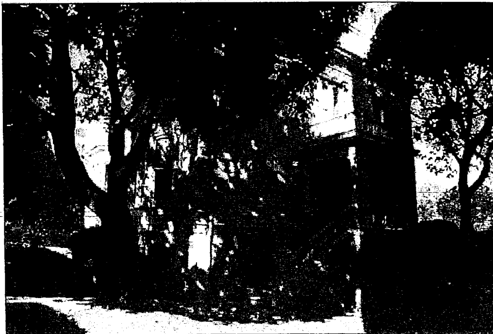
Photo 7. Burr House, 1772 Vallejo Street, 94123. Site, view northwest. Note mature trees planted adjacent to porch foundation and tree limbs encroaching on house
