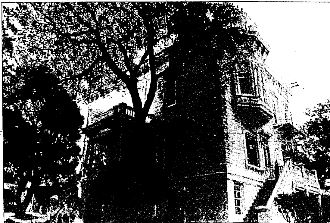
Photo 16. Burr House, 1772 Vallejo Street, 94123. East (left) and north (right) elevations, view southwest. Note mature trees encroaching on house.
