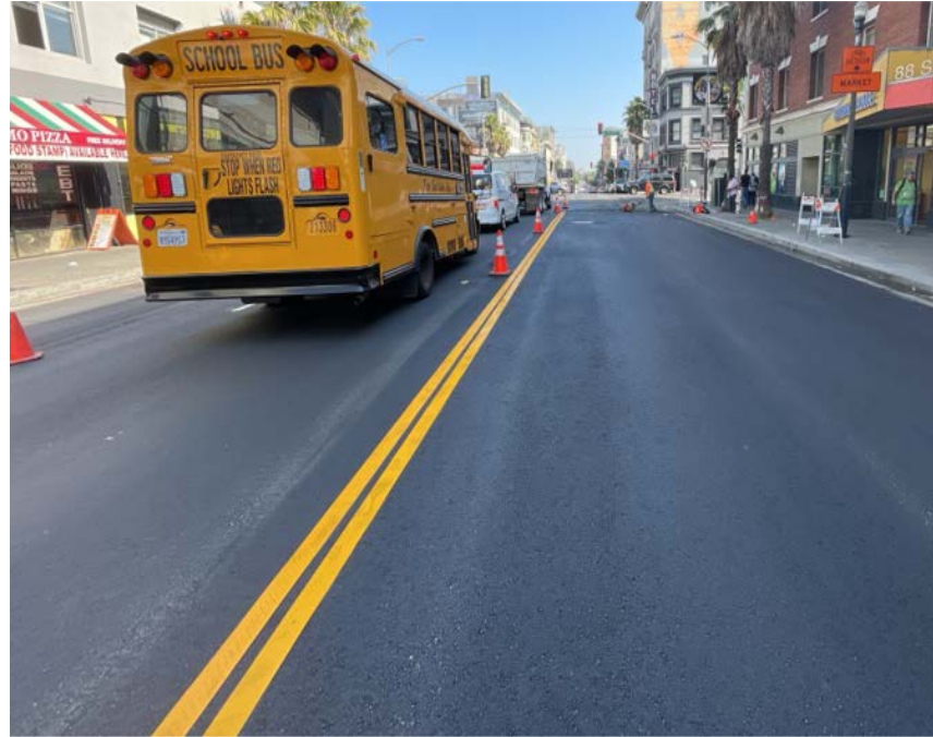
6th and Mission: New asphalt paving
