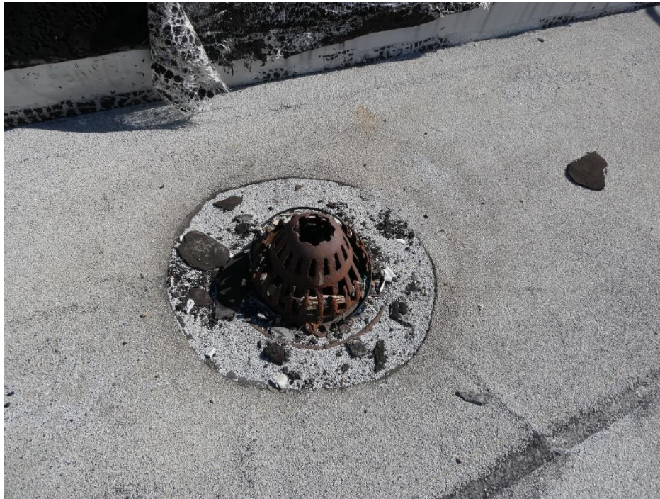
Figure 19: The drains appear to be partially or completely blocked with debris. It is unclear if any of the drains are functioning properly. (Page & Turnbull, 2024)
