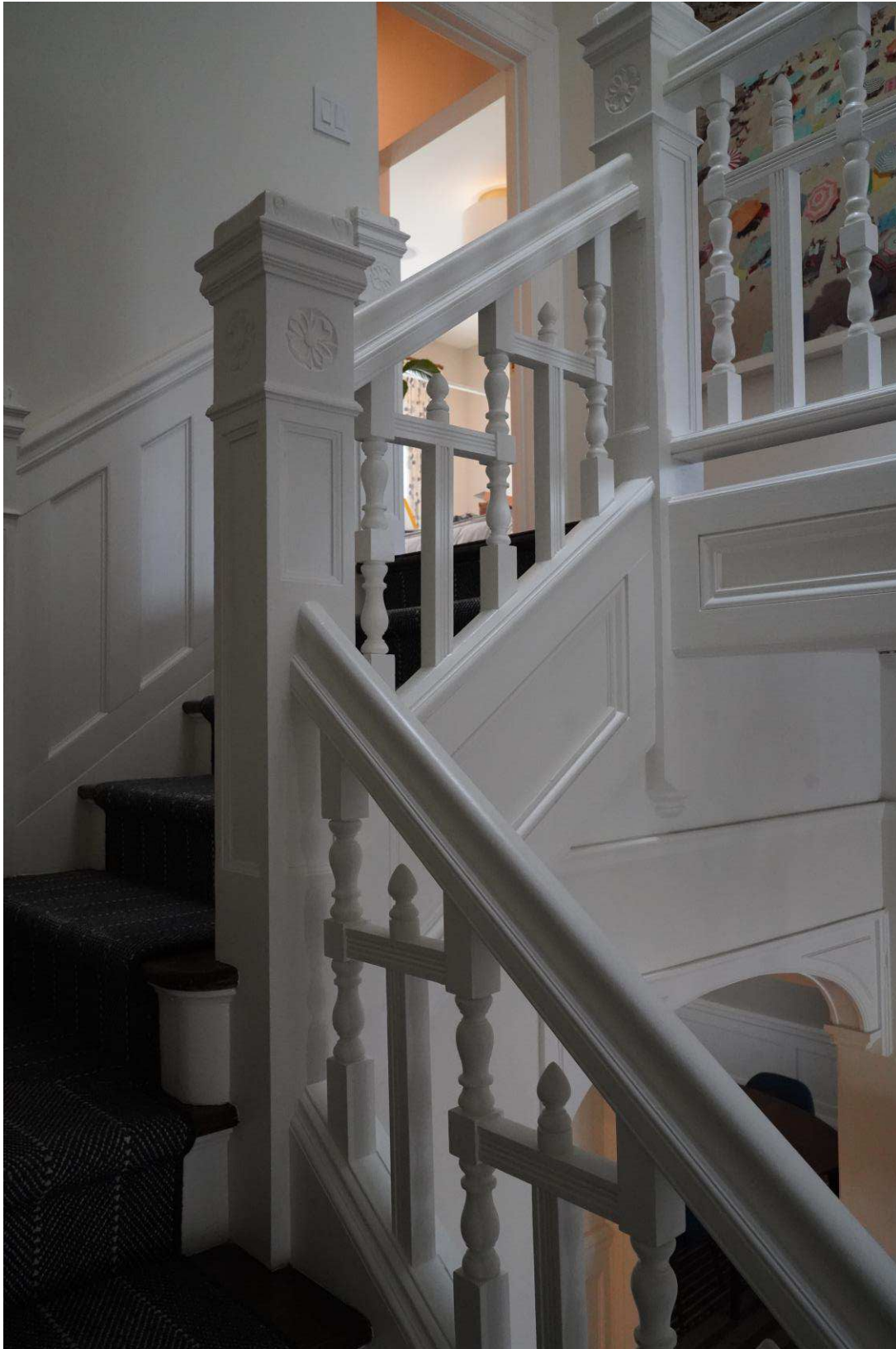
Figure 45. Detail of stair railing, view southwest.
