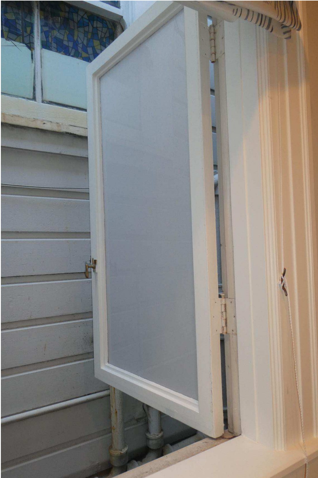
Figure 49: Non-historic casement sash at the second floor looking into the northeast lightwell.
