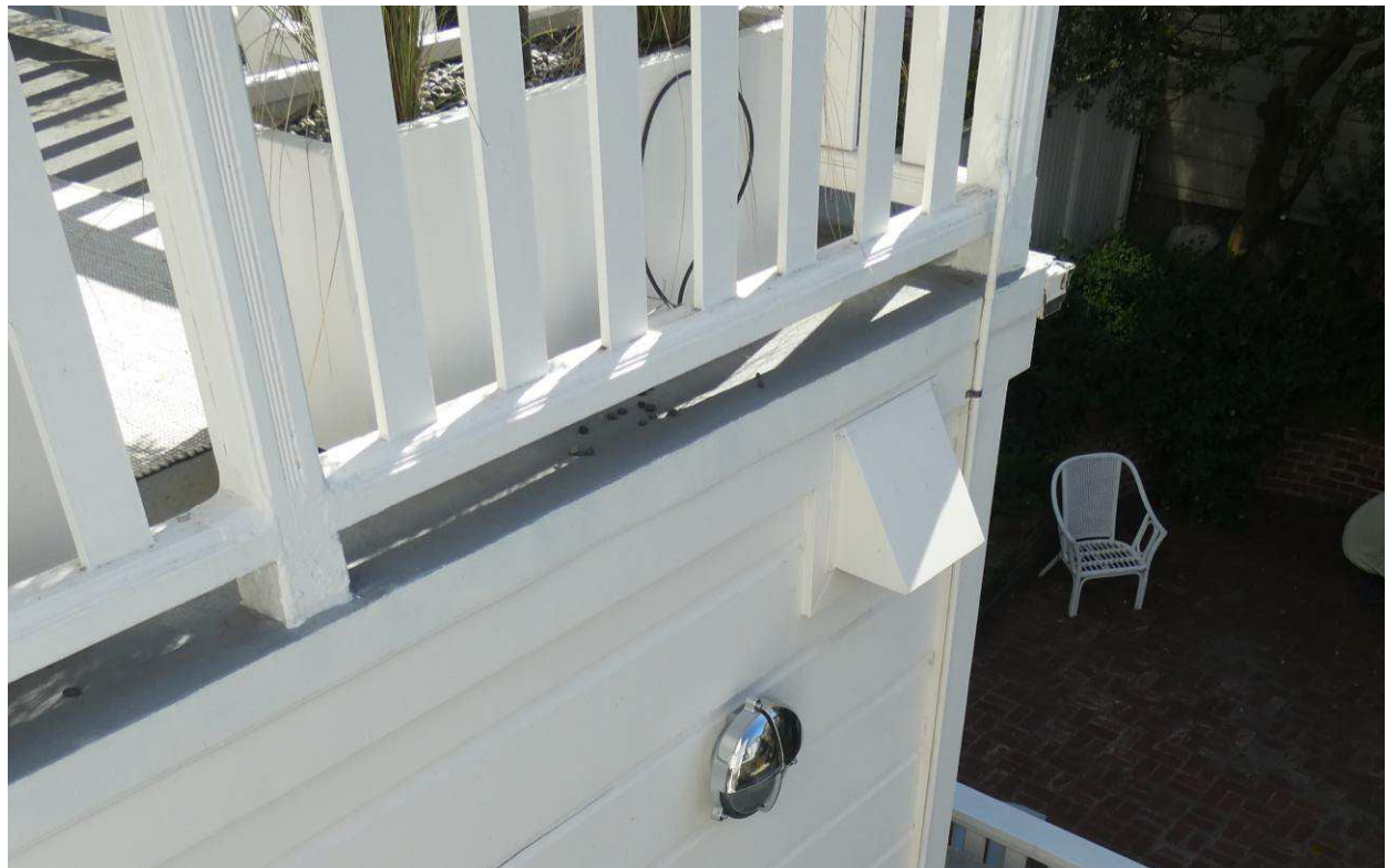
Figure 55: Detail showing the asphaltic roof at the decking above the first floor kitchen.
