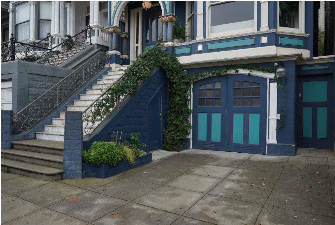
Figure 27. Garage and exterior front stairs at northwest facade, view southeast.
