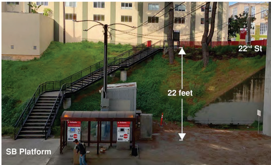
Southbound Platform Staircase
