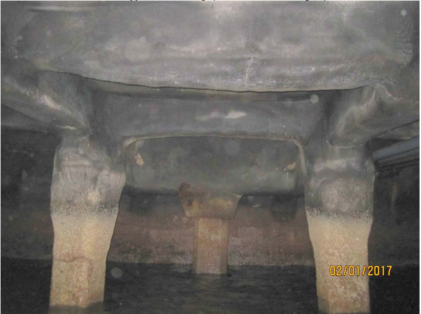
Photo 2. Typical condition of sea wall adjacent to Pier 9. No significant damage noted.
