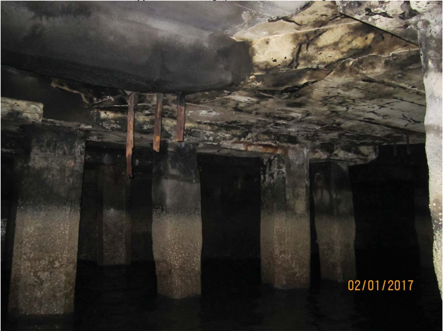
Photo 4. Northern rail track at upper right, concrete surface coated in waterproofing paper.
