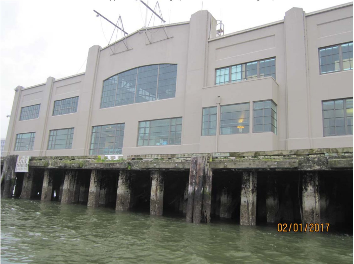
Photo 1. Outer end of pier
