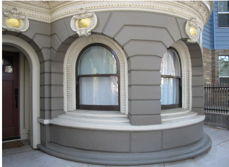
Figure 4: Ground level rounded bay base.
