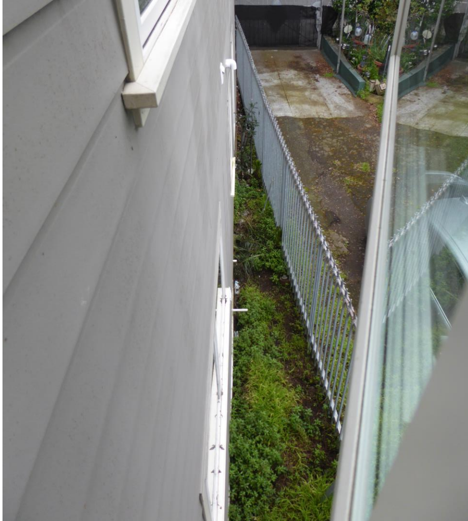
Figure 36: Inaccessible landscaped area adjacent to the north facade.
