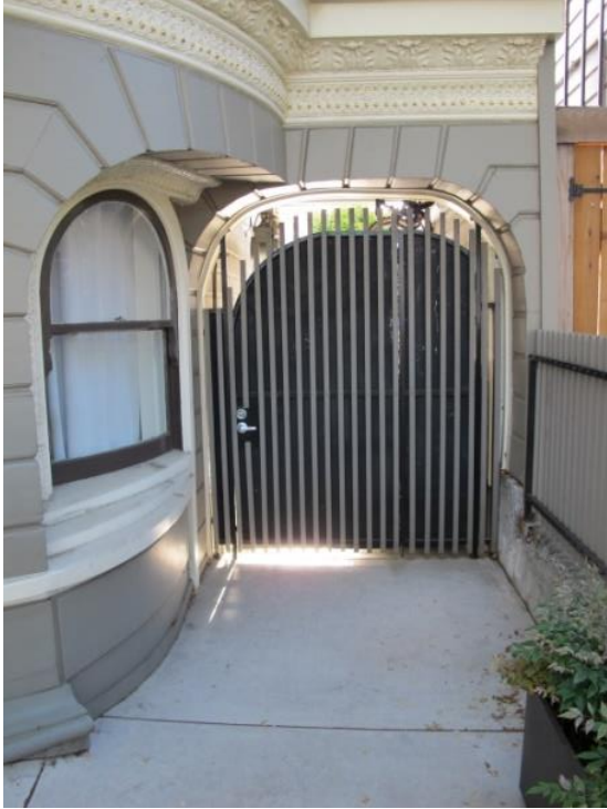
Figure 5: Security gate leading to south façade and backyard.
