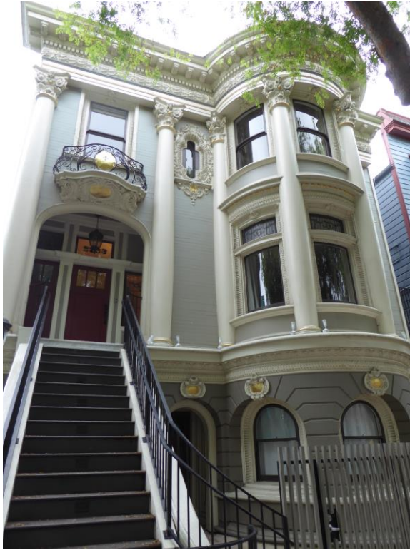
Photo 2: Front facade Looking east
