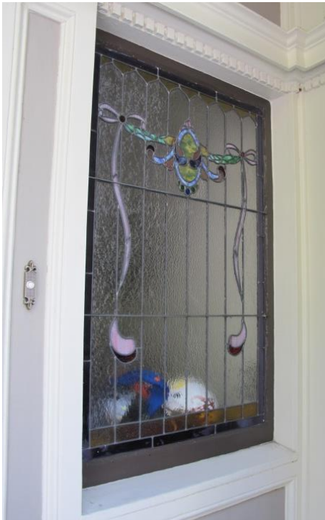
Figure 7: Fixed leaded stained glass window within entry area.
