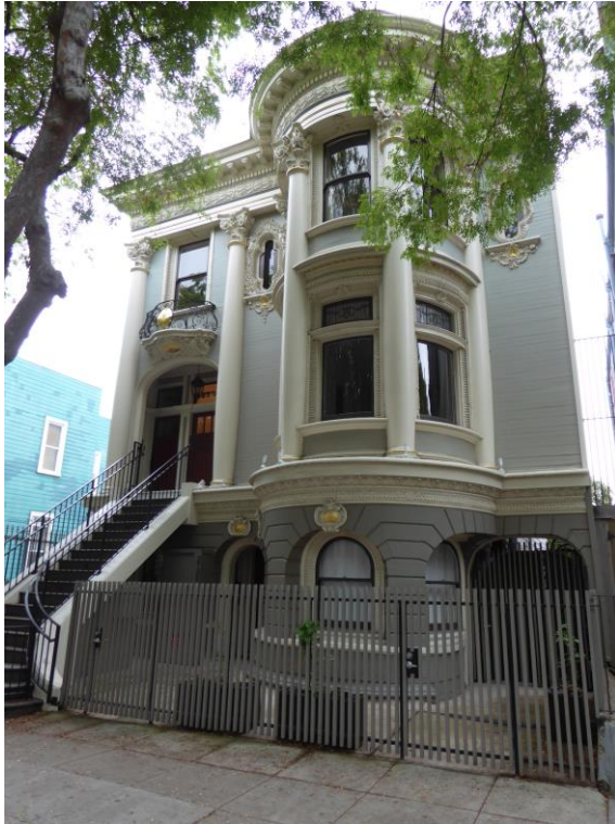
Photo 1: Front facade Looking northeast
