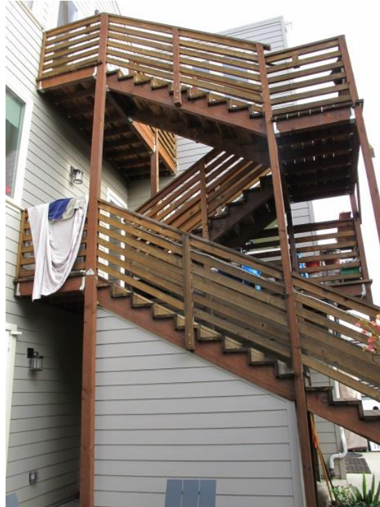
Figure 18: Exterior three-story stairs.
