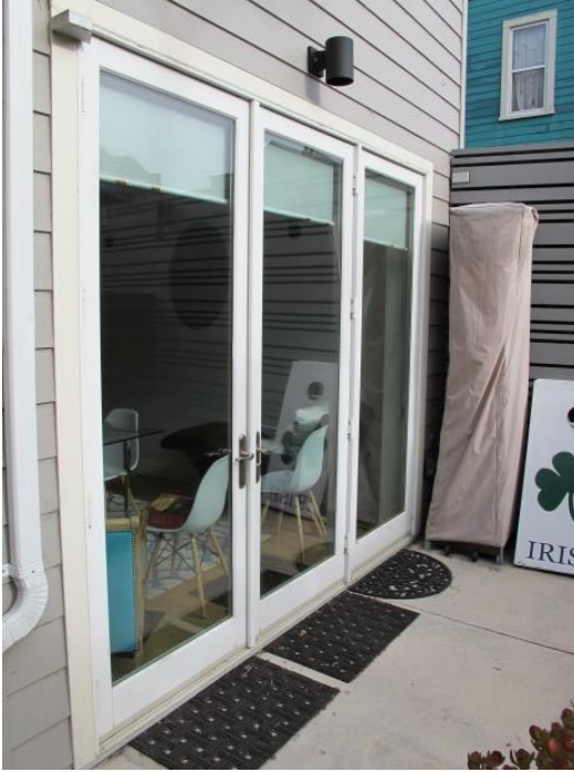
Figure 19: North side ground level.
