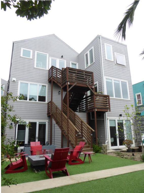
Photo 4: Rear facade Looking west
