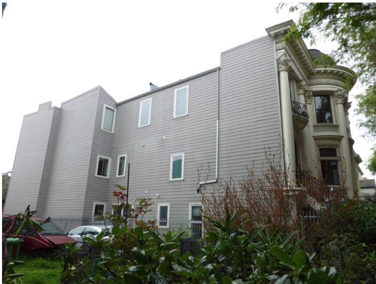
Photo 3: Side facade Looking south
