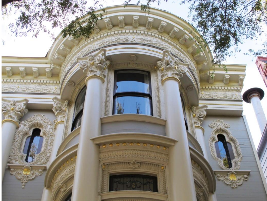
Figure 12: Bay flanked by oval windows in elongated quatrefoil surrounds (south window has a simpler surround).
