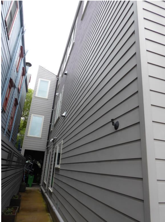
Photo 5: Side facade Looking west
