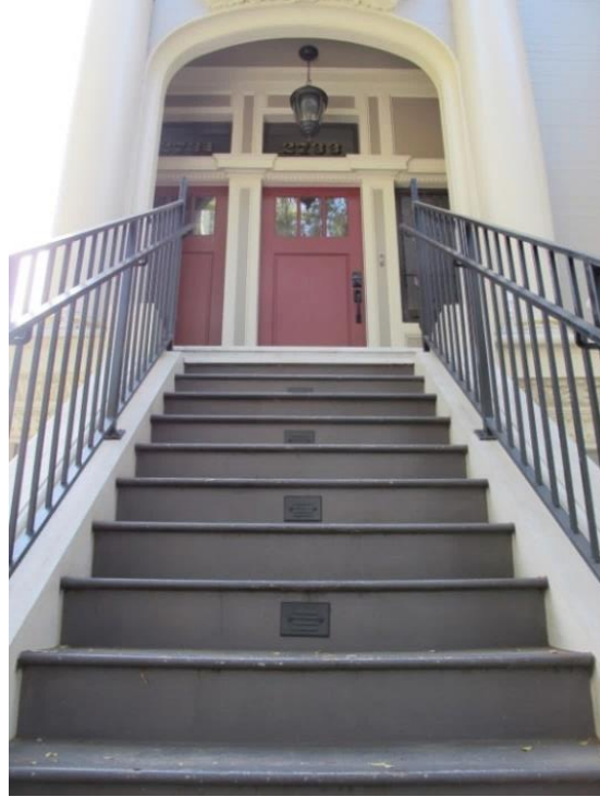
Figure 6: Exterior stairs leading to second story.
