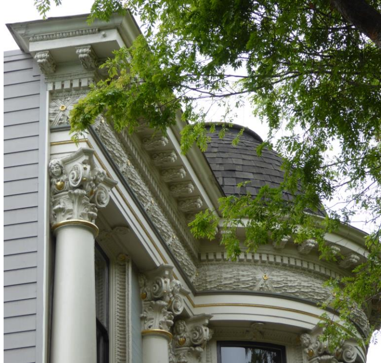
Figure 22: Detail of carved ornamental entablature, cornice, and column capitals.
