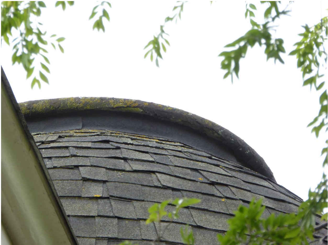
Figure 31: Detail of shingles at turret.
