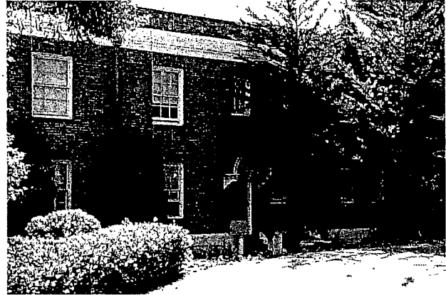
West elevation of south wing, April 2015
