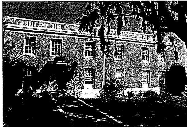
South elevation of south wing, April 2015
