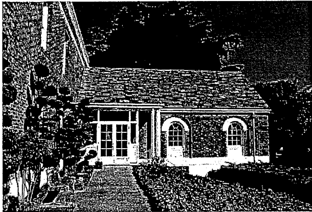
South elevation of chapel at north wing, April 2015
