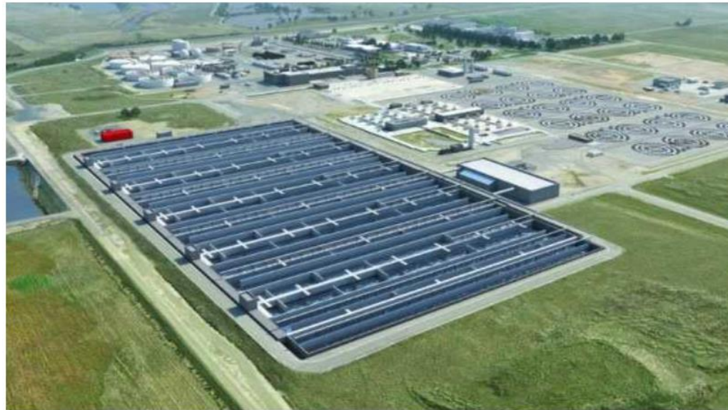
An artist rendering shows the planned biological nutrient removal facility planned for the Sacramento regional sewage treatment plant in Elk Grove. SOURCE: Courtesy: Sanitation District
