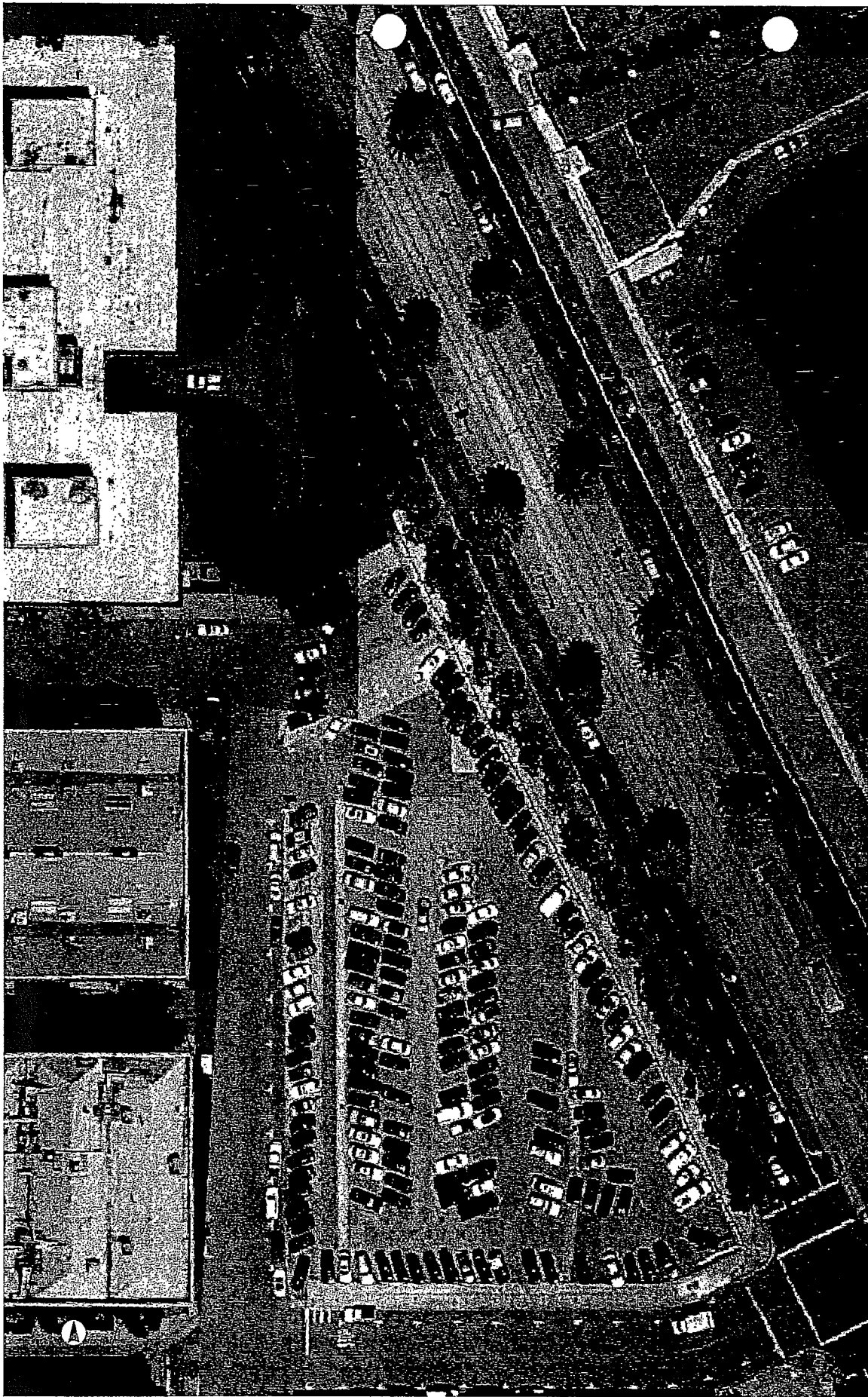
FIGURE 15 AERIAL VIEW OF THE EMBARCADERO: UNION TO JUST SOUTH OF GREENWICH STREET
