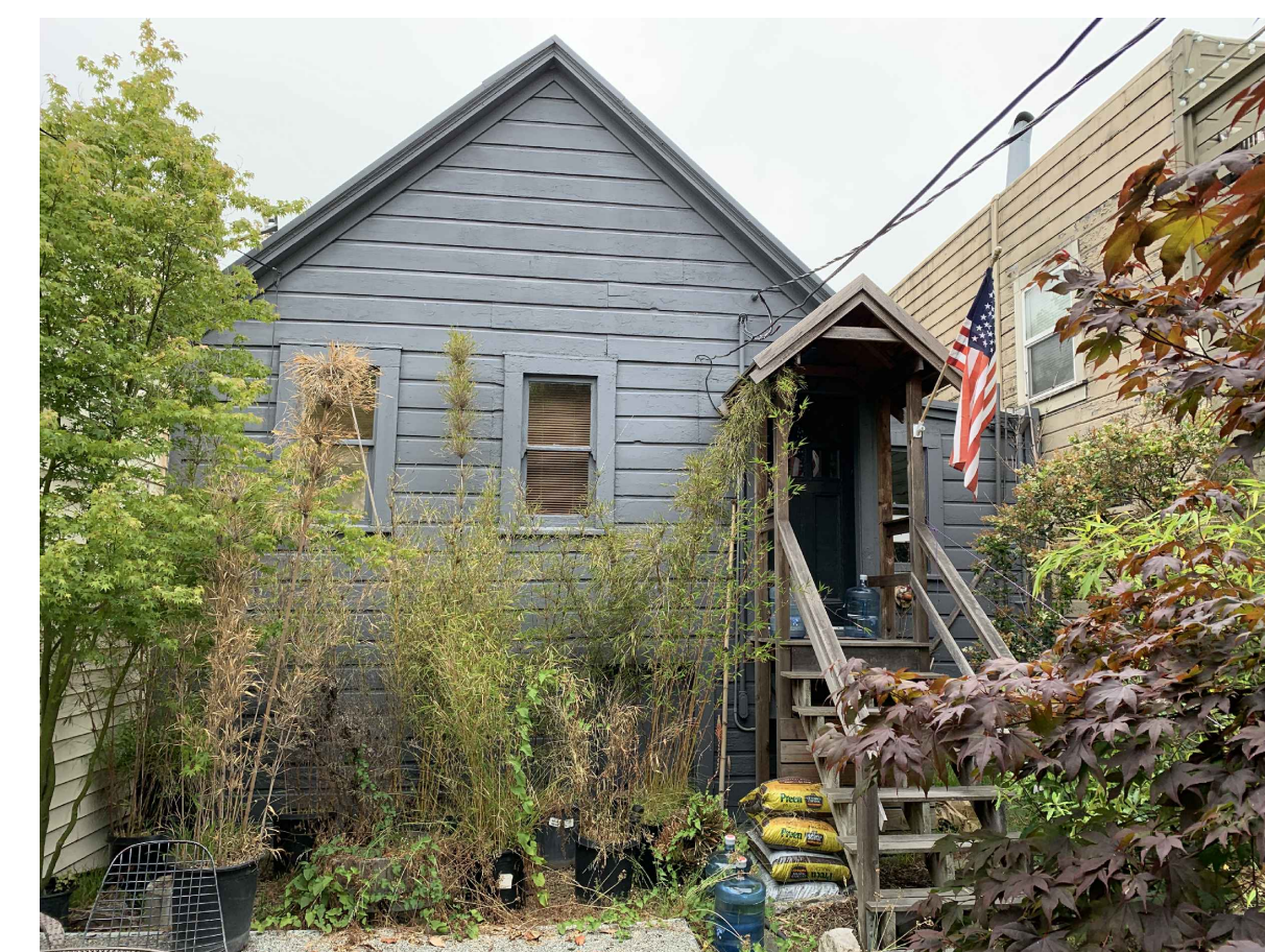
FRONT VIEW: FROM FRONT YARD
