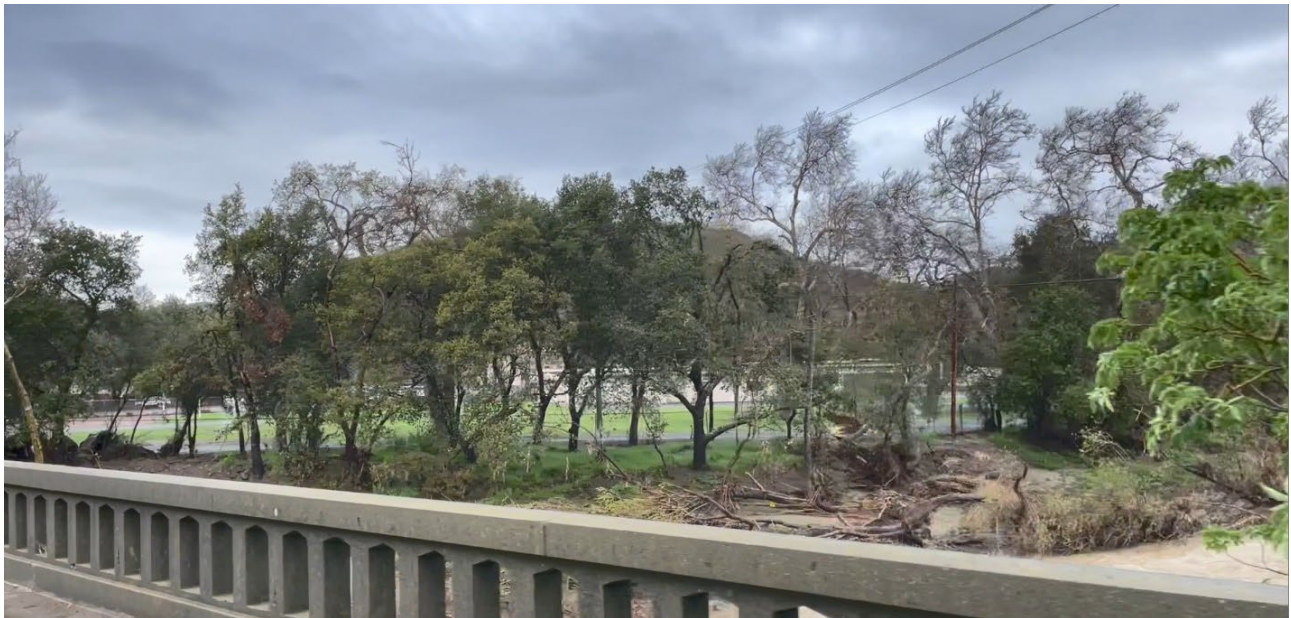
Figure 5: View of the Creek Crossing Work Area Traveling Westbound on Niles Canyon Road
