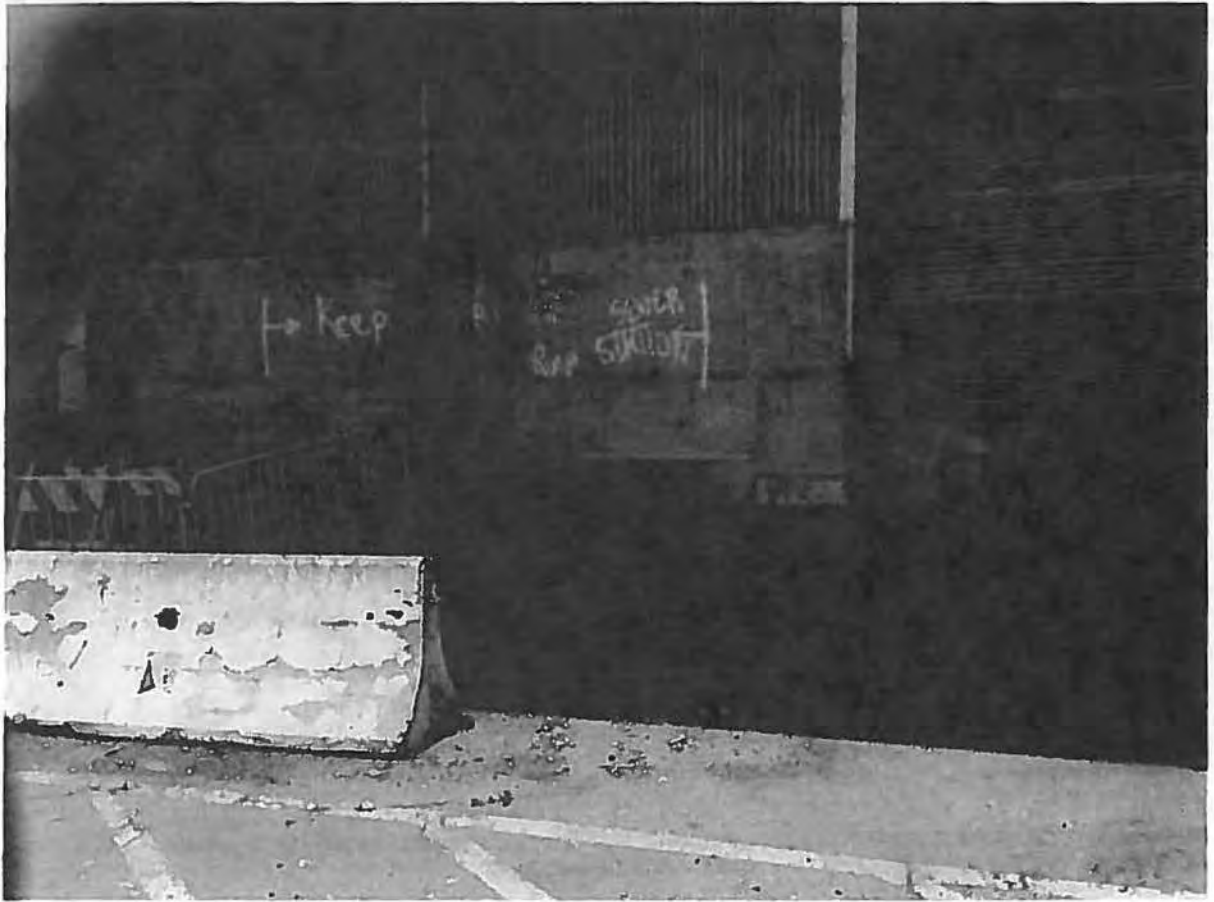
P80 A Shed Sewer Pump Station (Image #2)
