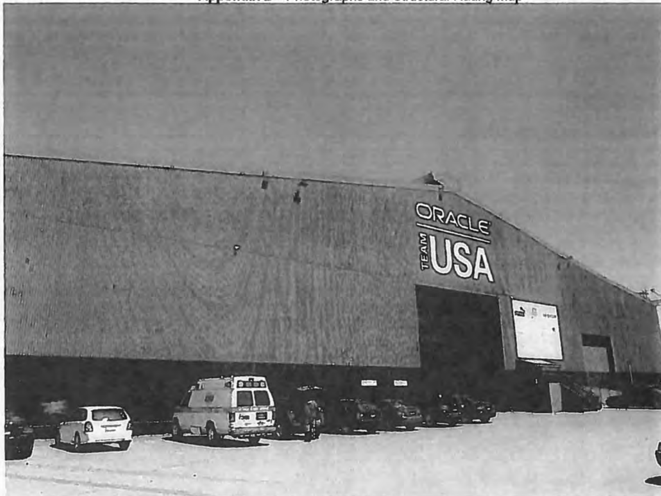
Photo 1. View of the west elevation
