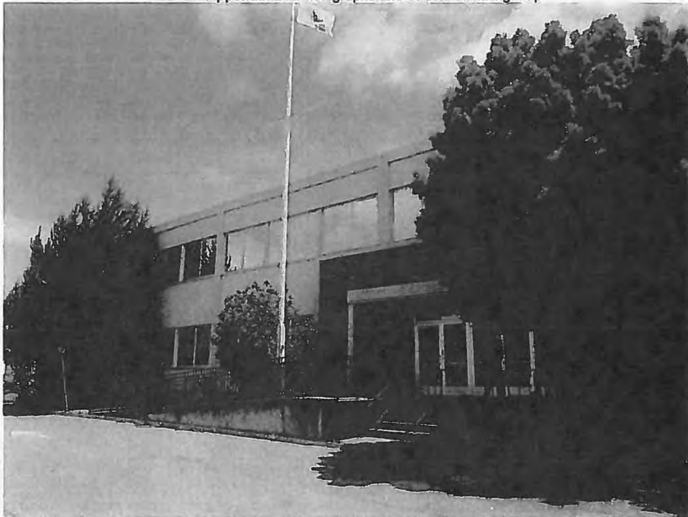
Photo 4. View of the west elevation
