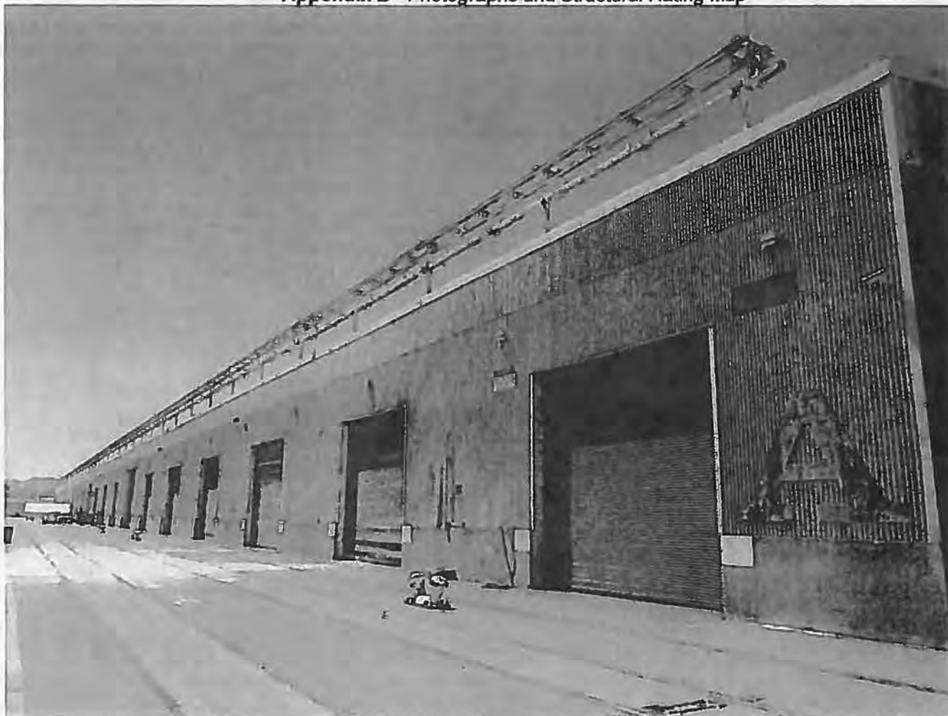
Photo 13. View of the south elevation
