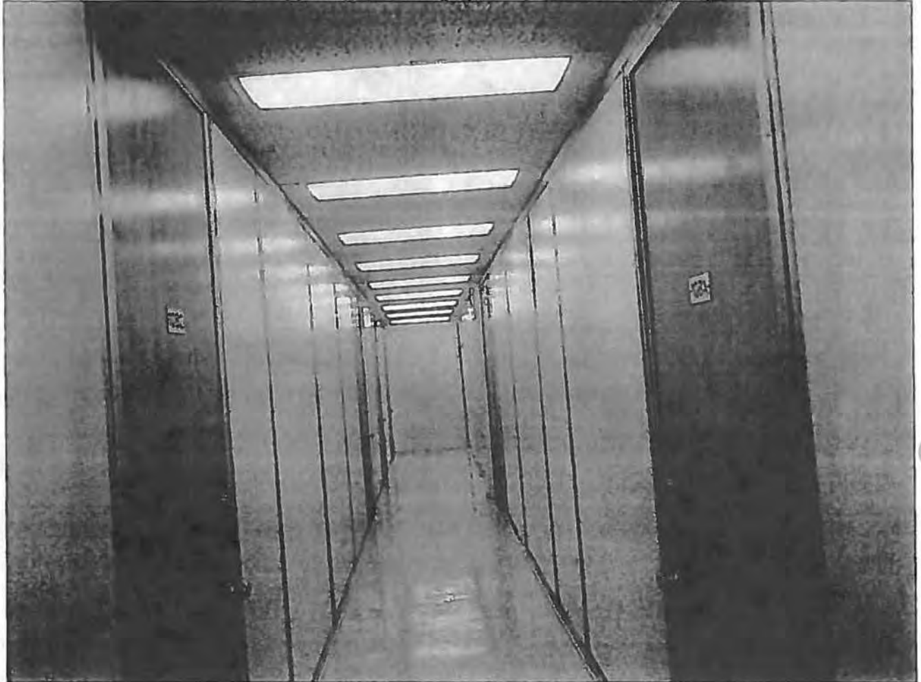
Photo 9. View of the interior first floor hallway
