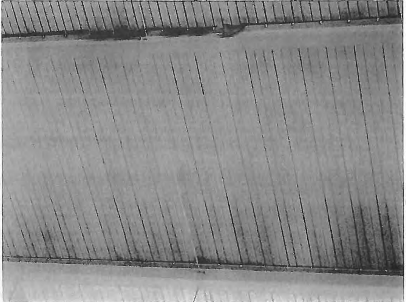
Photo 9. View of the underside of the roof deck
