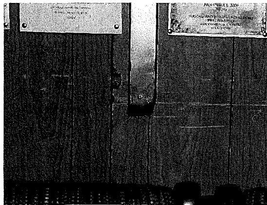
Figure 16: Ends of gold crucifix have missing paint. Wood paneling has abrasion marks from furniture.
