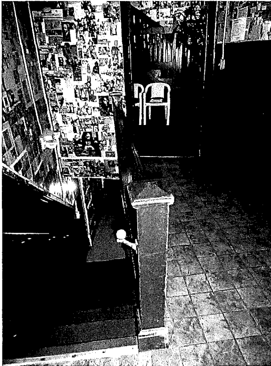
Figure 23: General wear and tear of collage and wood stair railing from pedestrian traffic.
