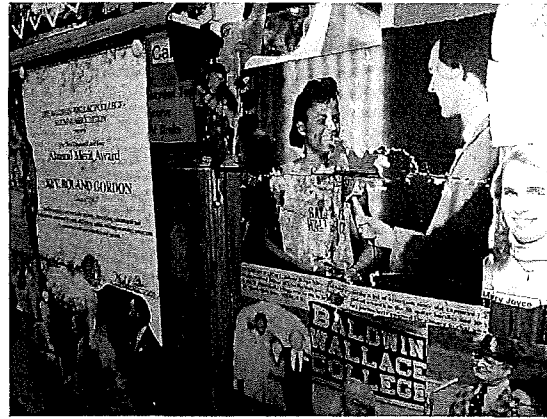
Figure 22: Displacement and movement of wood paneling resulting in attached collage to tear.
