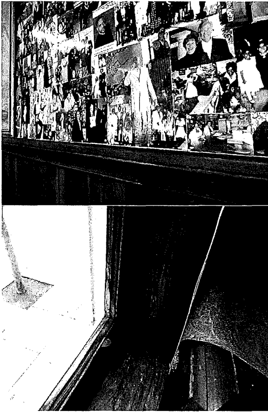
Figure 11: College comprised of photos is faded due to UV-light related deterioration. Pedestrian traffic has abraded some of the photos and wainscoting.
