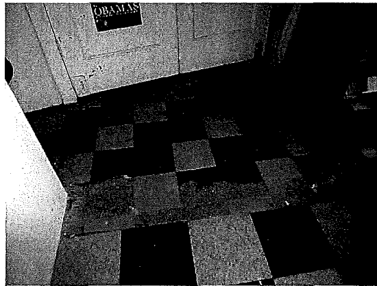
Figure 28: Exposure of multiple layers of flooring.
