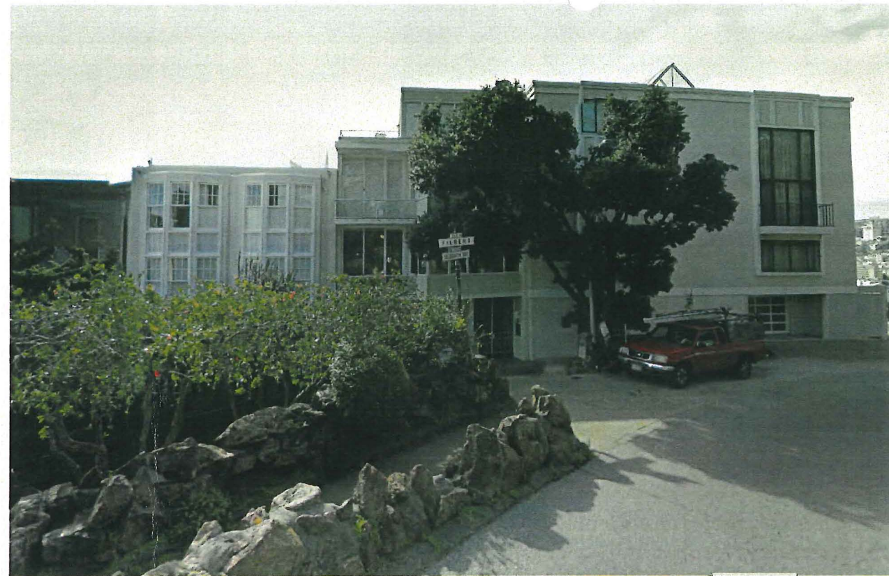
6 ADJACENT CONTEXT TO EAST OF SUBJECT PROPERTY SCALE: 1:0.96
