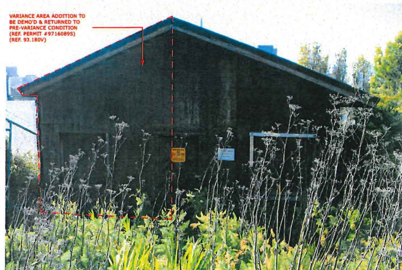
1 COTTAGE: EXISTING NORTH FACADE NOT TO SCALE
