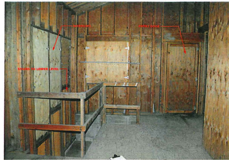
6 COTTAGE: EXISTING UPPER LEVEL LOOKING NORTH NOT TO SCALE
