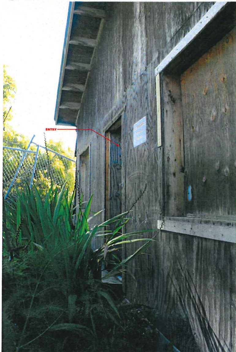
4 COTTAGE: EXISTING NORTH FACADE NOT TO SCALE
