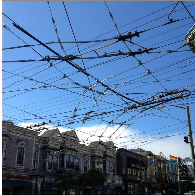
Figure 69 Example of complex overhead wire arrangement, Castro District (Source: Google Street View)
