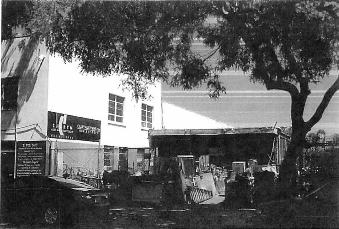
Figure 11: South facade, facing northeast.
