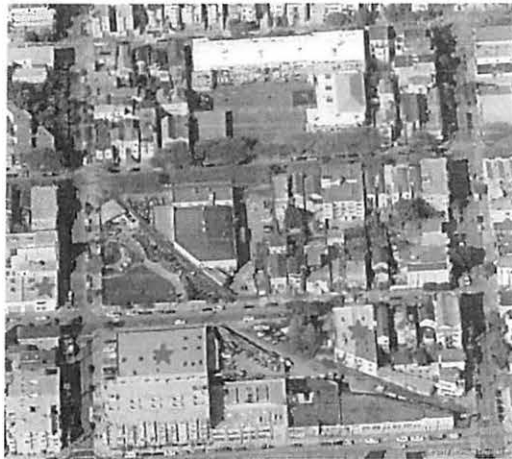
Figure 17: Aerial photograph of 2675 Folsom Street (outlined in red) and surrounding area. Light industrial buildings are indicated by red stars. The diagonal trace of the defunct rail line can be seen rising from right to left. Cesar Chavez Elementary School is the large building at top center. The remainder of buildings are residential. North is to the right. Source: Bing Maps, edited by author.
