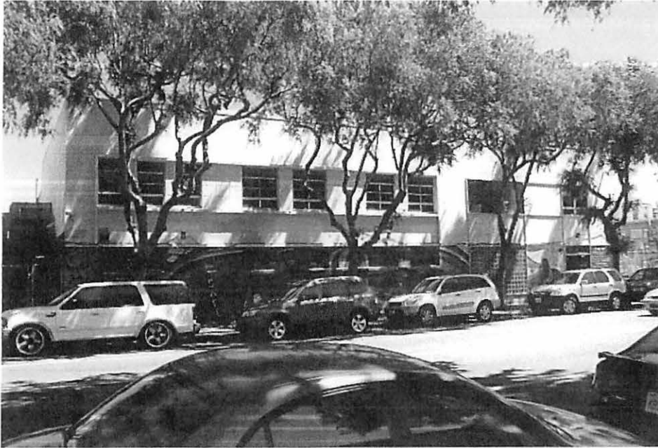
Figure 3: Primary (west) facade, facing southeast.
