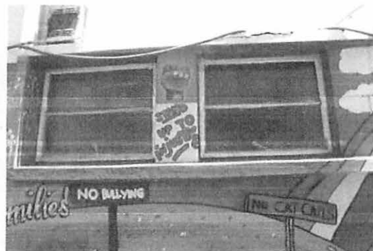
Figure 5: First story windows and portions of the 2012 mural, facing east.
