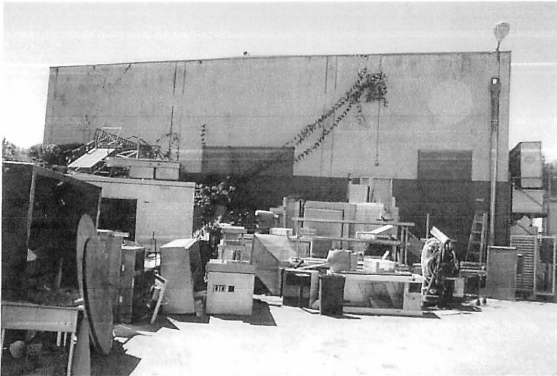
Figure 14: Rear (east) facade, facing west.
