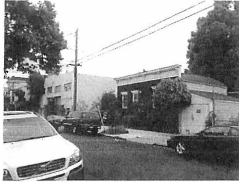
Figure 28: 935 Treat Avenue (at left) facing northeast.
