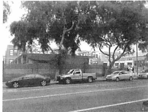
Figure 26: Rear facade and play yard of Cesar Chavez Elementary School, west side of Folsom Street between 22 nd and 23 rd streets, facing northwest.
