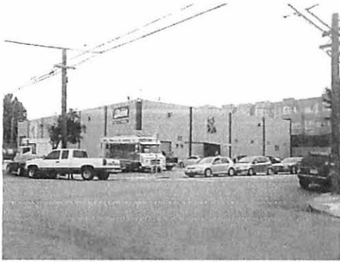
Figure 27: 3050 23rd Street, facing northeast.
