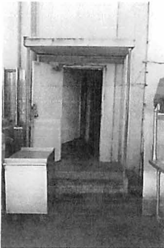
Figure 9: North facade entrance, facing south.
