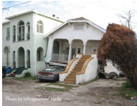
The result of a soft story collapse.
