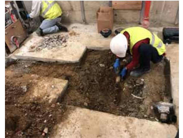
Mission Cultural Center for Latino Arts Elevator Work
