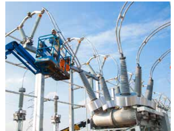
Warnerville Substation Rehabilitation
