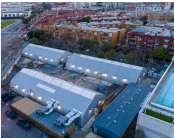
Embarcadero SAFE Navigation Center
