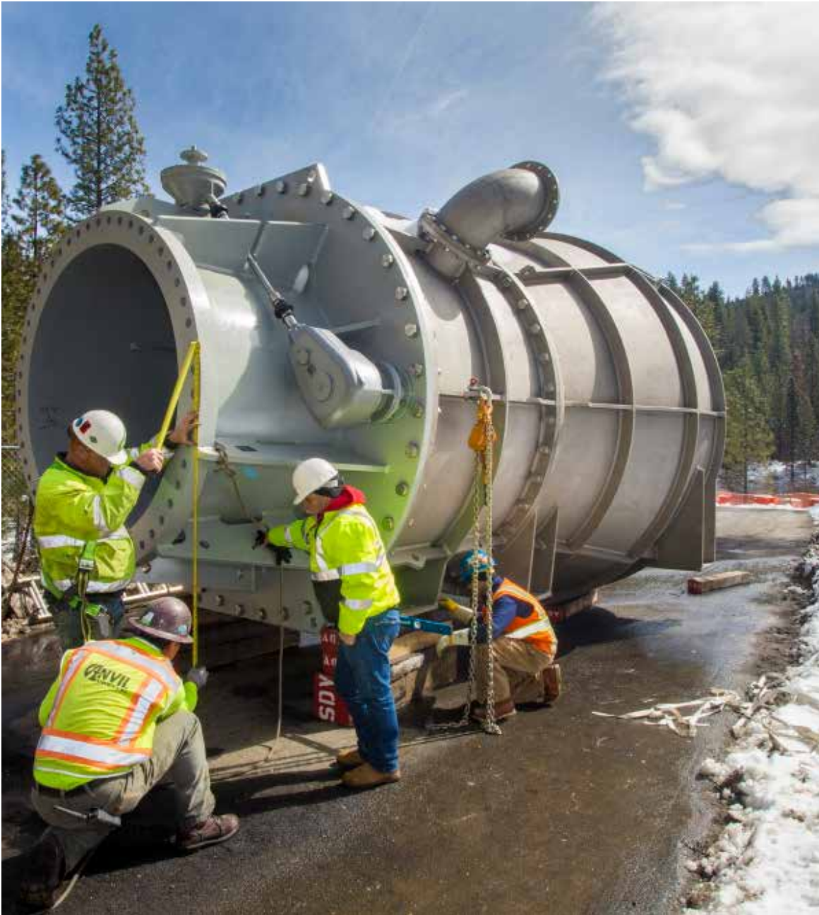
Cherry Dam Outlet Works Rehabilitation
