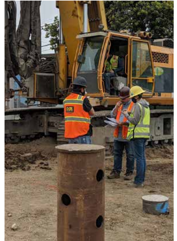
Construction at Maxine Hall Health Center
