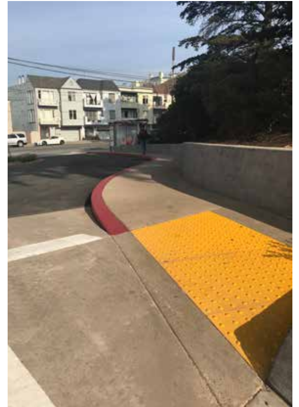
New Curb Ramp
