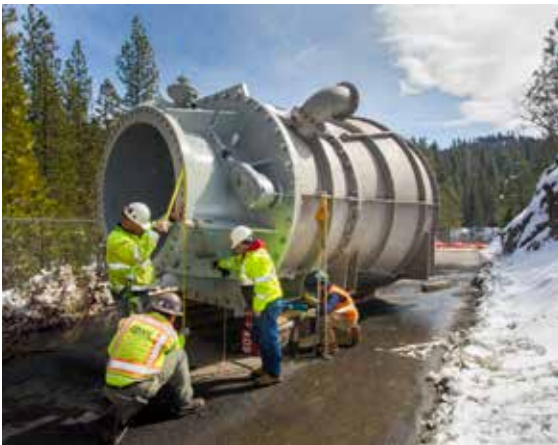
Cherry Dam Outlet Works
