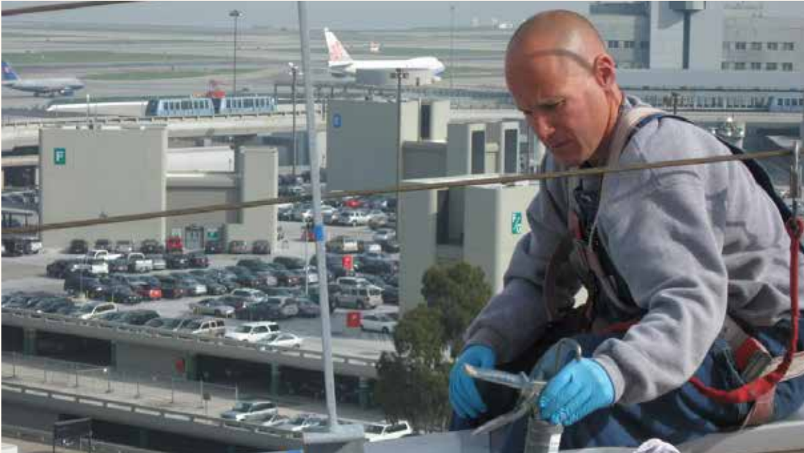
Roof Repair at SFO
