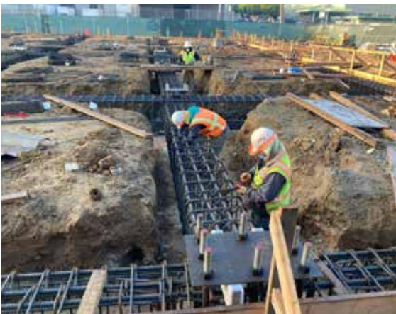
Construction at South East Health Center
