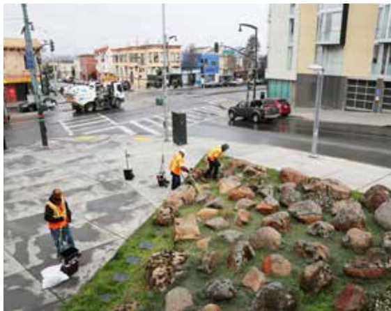
Bayview Streetscape Work
