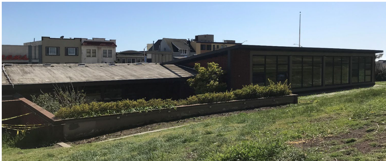
Parkside Branch Library, north elevation, view southwest, 2023. Source: San Francisco Planning Department
