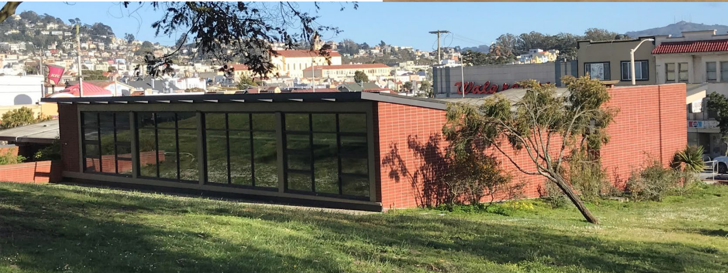
Parkside Branch Library, north and west elevations, 2023 Source: SF Planning Department
