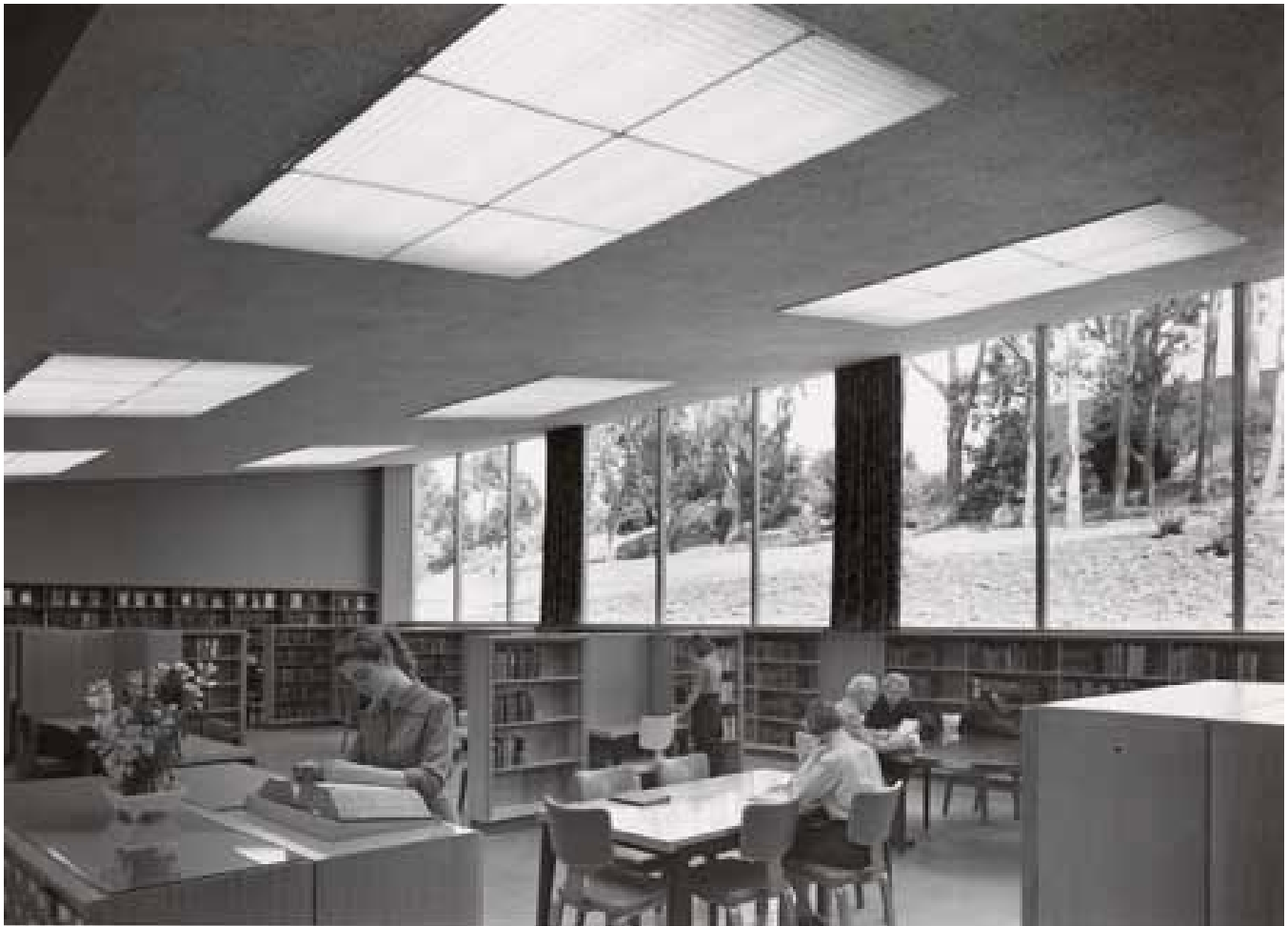
Parkside Branch Library, interior, view northwest, circa 1951.
