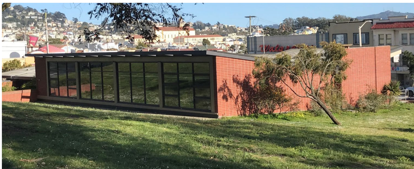
Parkside Branch Library, north elevation, view southeast, 2023. Source: San Francisco Planning Department
