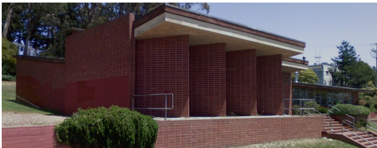
Parkside Branch Library, front and west elevations, view northeast, 2008.
