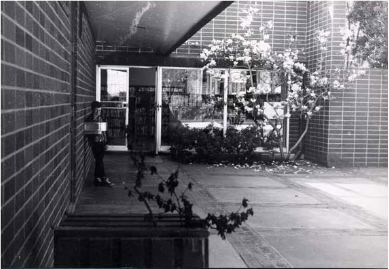
Parkside Branch Library, terrace, view west, 1970.
