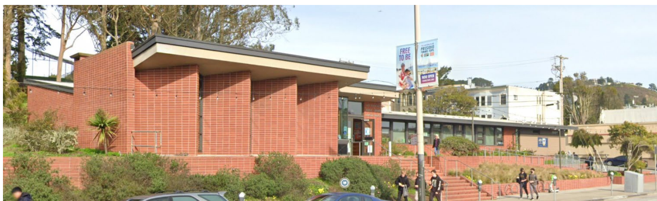
Parkside Branch Library, front façade, view northeast, 2023. Source: Google Streetview
