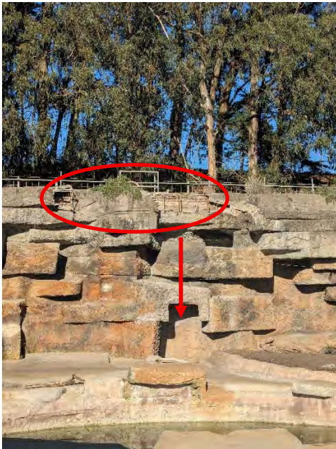
Exhibit 4.9: Examples of Infrastructure of Concern
