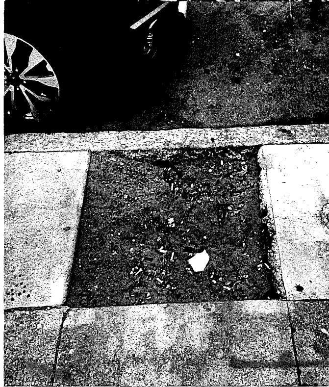
Maintenance funding limits planting
