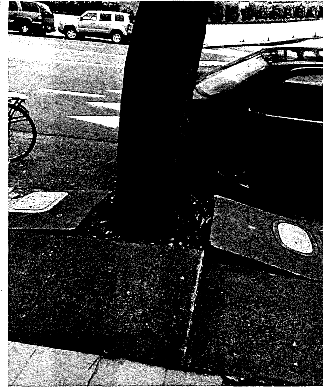
Sidewalk repair needs
