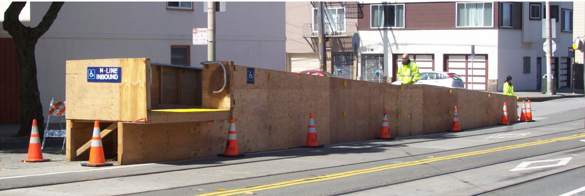
Example of a temporary accessible ramp
