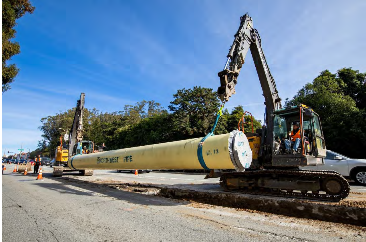
New pipe for Potable Emergency Firefighting Water Systems pipeline at 19th Ave and Sloat Blvd.
