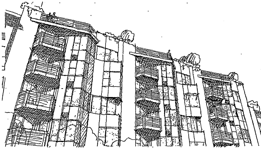
ILLINOIS STREET PARAPET
