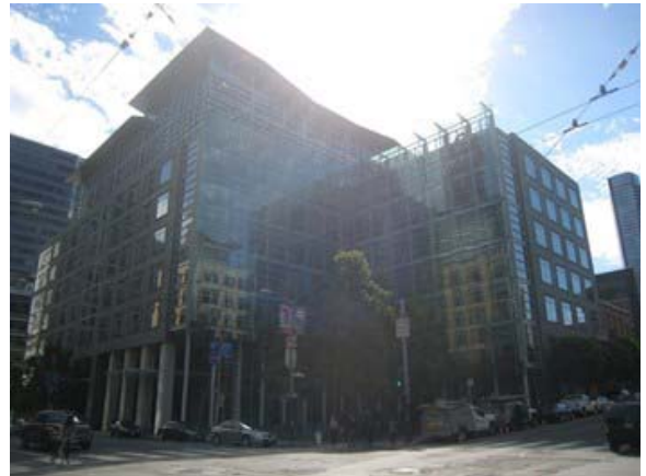
Lease 4 Foundry Square II
