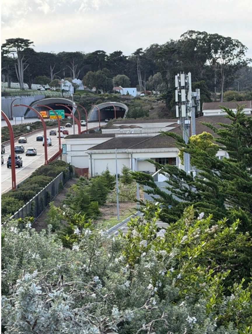
130 foot monopole located in the parking lot of Sports Basement adjacent to 101
