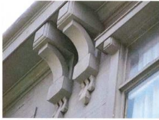
Detail of cornice brackets
