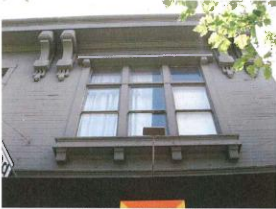
Detail of window and cornice
