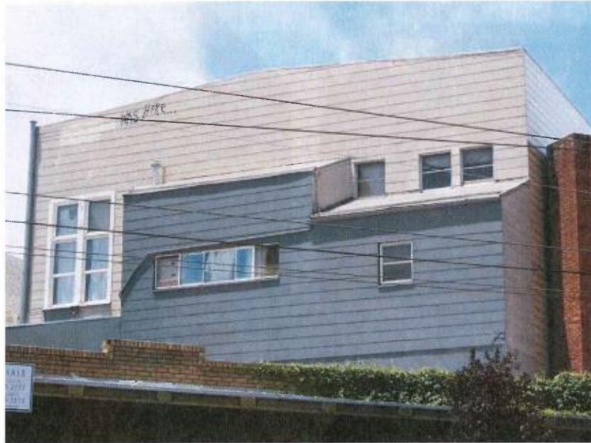
View of the rear elevation from Church Street.
