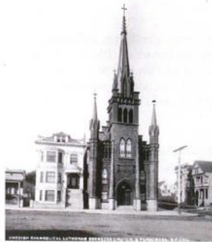
Ebenezer Swedish Lutheran Church and rectory, designed by August Nordin and completed in 1903. (San Francisco Public Library Historical Photograph Collection, AAB-1410)
