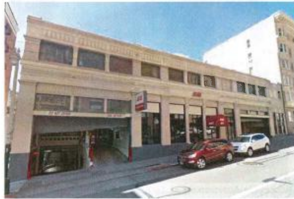
Cristobal Apartments at 750 O'Farrell Street (1913) at top; Parking garage at 675 Post Street (1919) at bottom. Both buildings incorporate a Greek key ornamental motif. (Google Maps)
