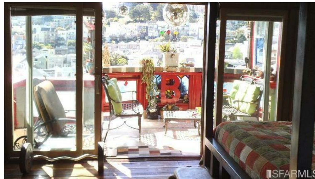
VIEW OF THE TOP FLOR REAR BALCONY NOTE THE APPROX. 36" HIGH RAILING AND THE DISCO BALLS HANGING FROM THE ILLEGAL REAR ROOF ANWING THAT WAS REMOVED
