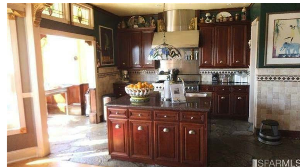
VIEW OF EXISTING BREAKFAST NOOK SEE CU10.5 FOR LARGER VEIV OF SIDE TRIANGLE
