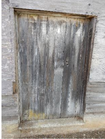
Figure 8. Greenhouse entrance door.
