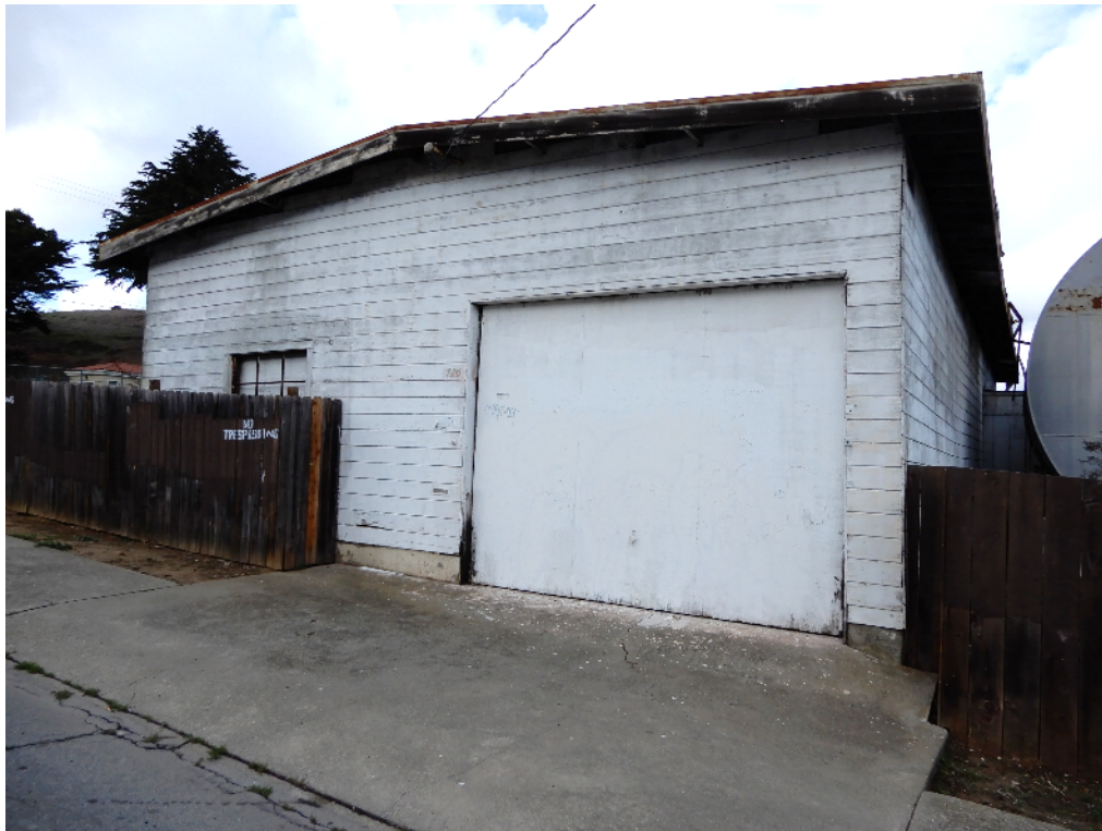
Figure 13. Office building, primary (south) façade, view facing northwest.
