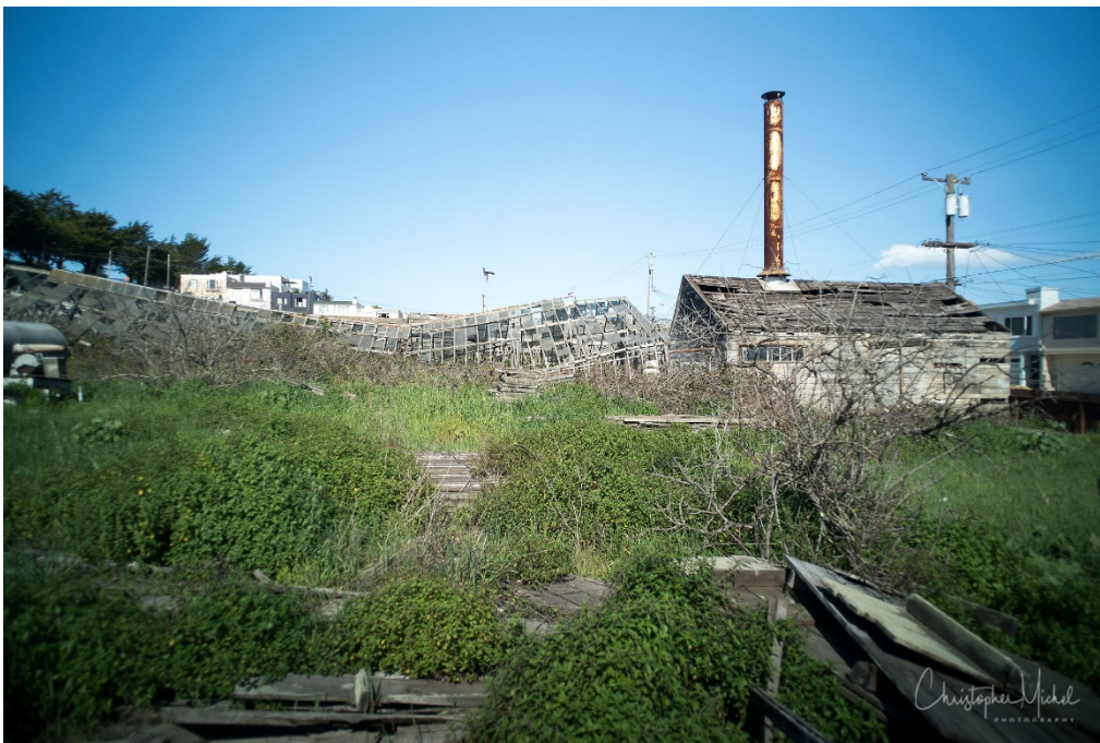
Figure 16. Open space at the southeast corner of the lot, view facing north. Courtesy of Christopher Michel Photography.
