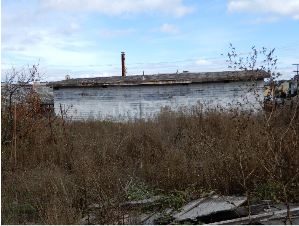
Figure 14. Office building, west façade, view facing east.
