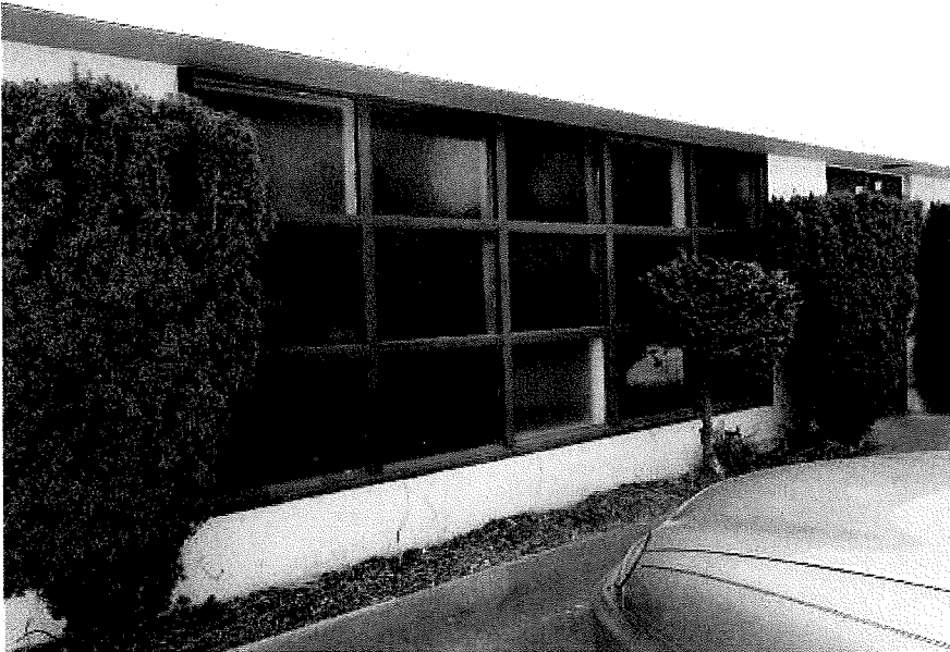
Multi-lite, wood sash windows with textured yellow glass at first floor, near northwest corner of north façade, view southwest.
