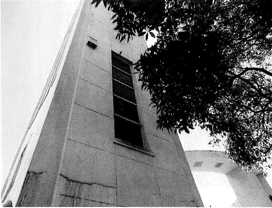
Detail of vertical wooden ribbon windows on bell tower. View southwest.
