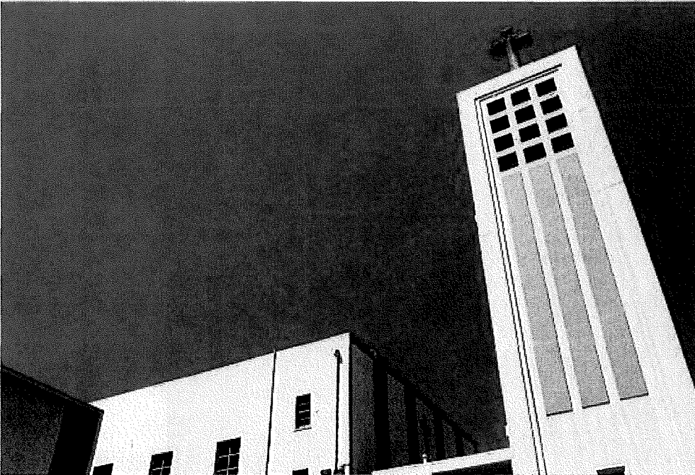
Upper portion of bell tower illustrating decorative scored borders, raised vertical bands, square voids, and cross ornament. View west.
