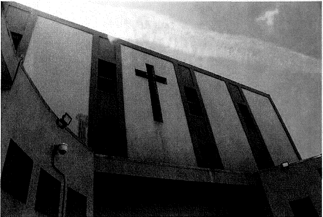
Detail of cross-shaped window on primary (north elevation) of main sanctuary building. View southwest.
