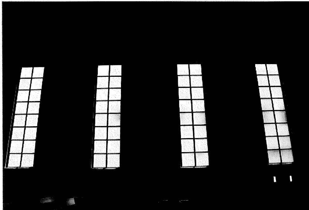
Vertical wood sash ribbon windows with divided lites and yellow glass, east interior wall.
