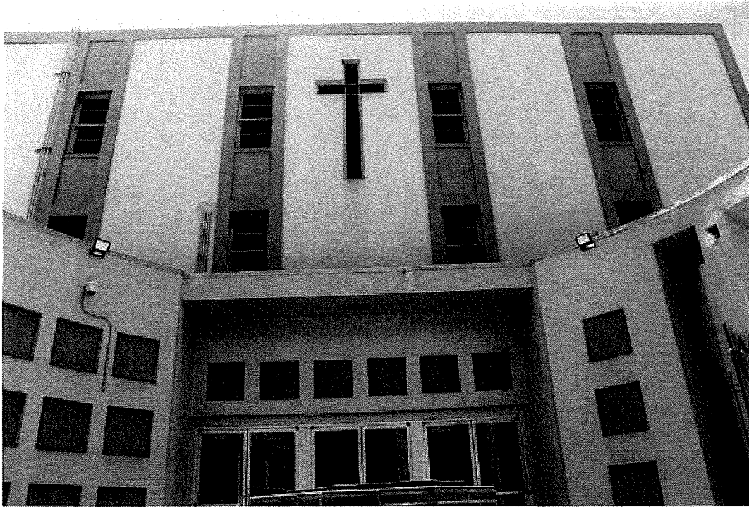
Primary (north elevation) of main church building. View south.
