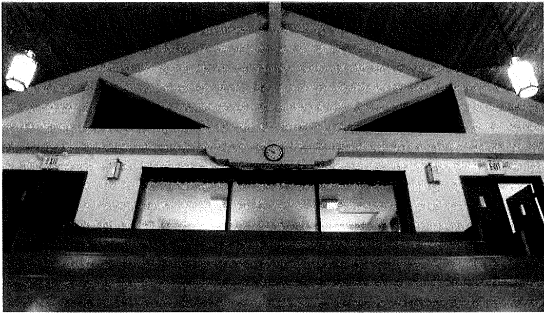
Mezzanine. View north.
