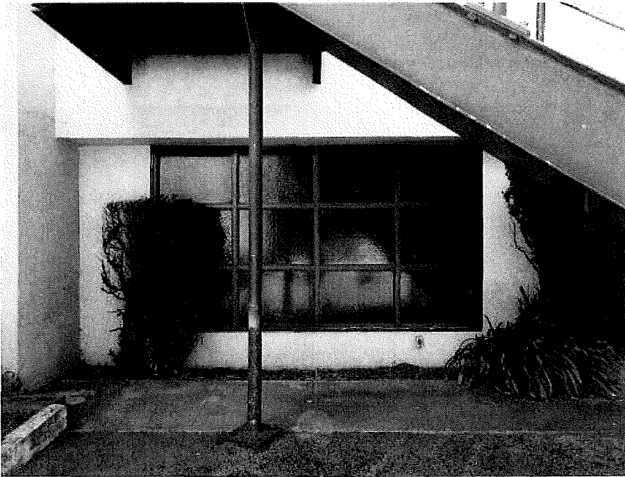
Multi-lite, wood sash windows with textured yellow glass at first floor. Northeast corner of north façade. View south.
