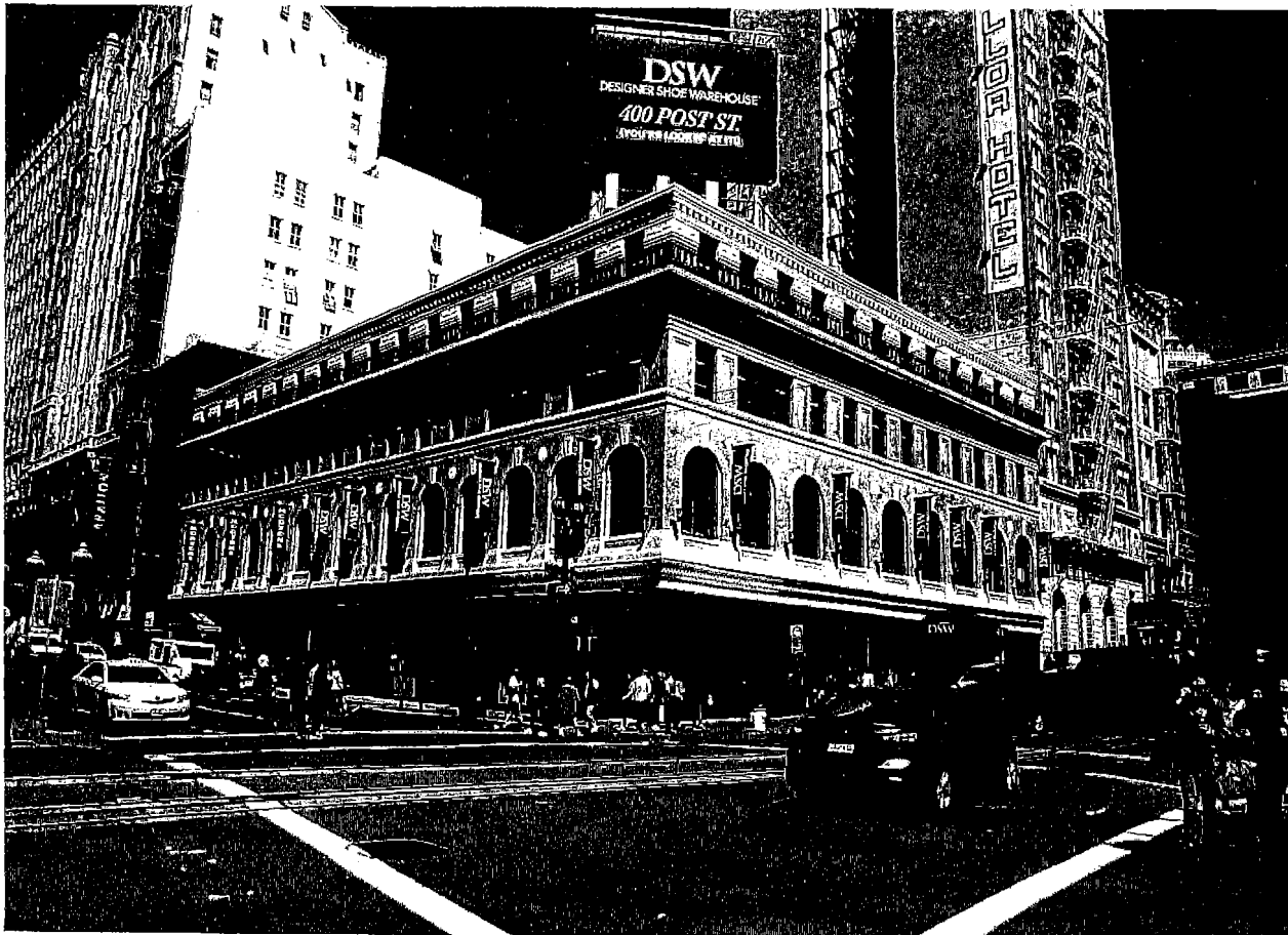
C. 400 & 421 Powell Street at the corner of Powell and Post streets (0296/006, built 1909). Source: Page & Turnbull
