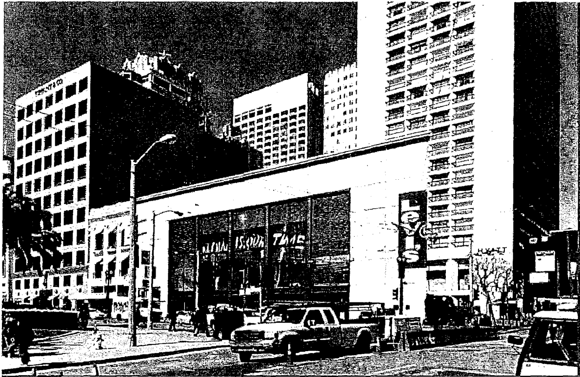
300 Post Street/345 Stockton Street
