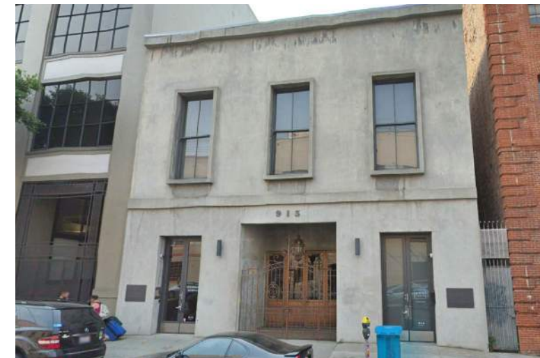
PROJECTED WINDOW FRAME WITHIN DISTRICT 915 Battery St.
