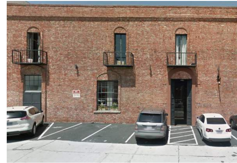
OFFSET WINDOWS EXAMPLE WITHIN DISTRICT 915 Front St.
