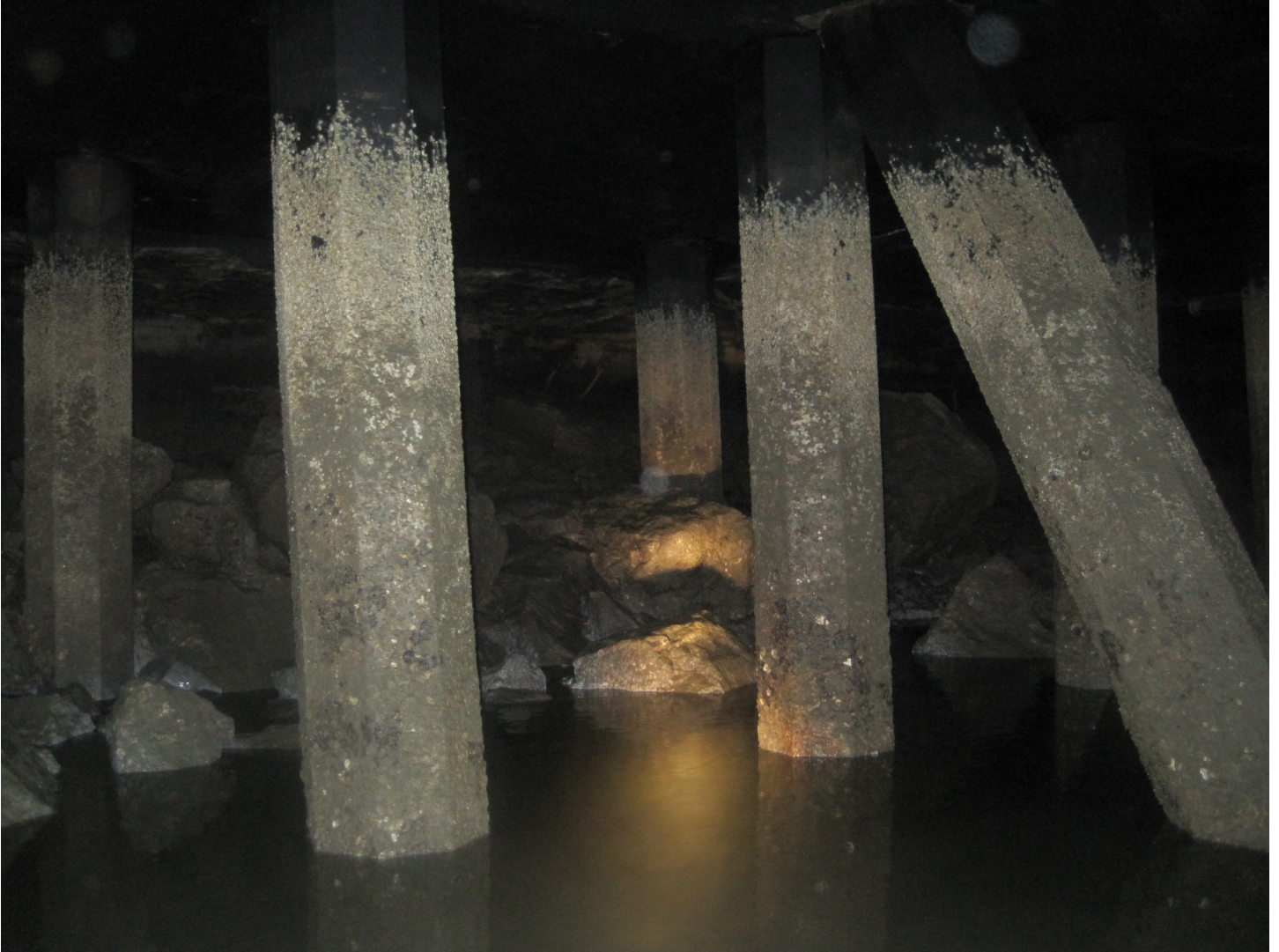
Photo 7. Seawall protected by rip-rap
