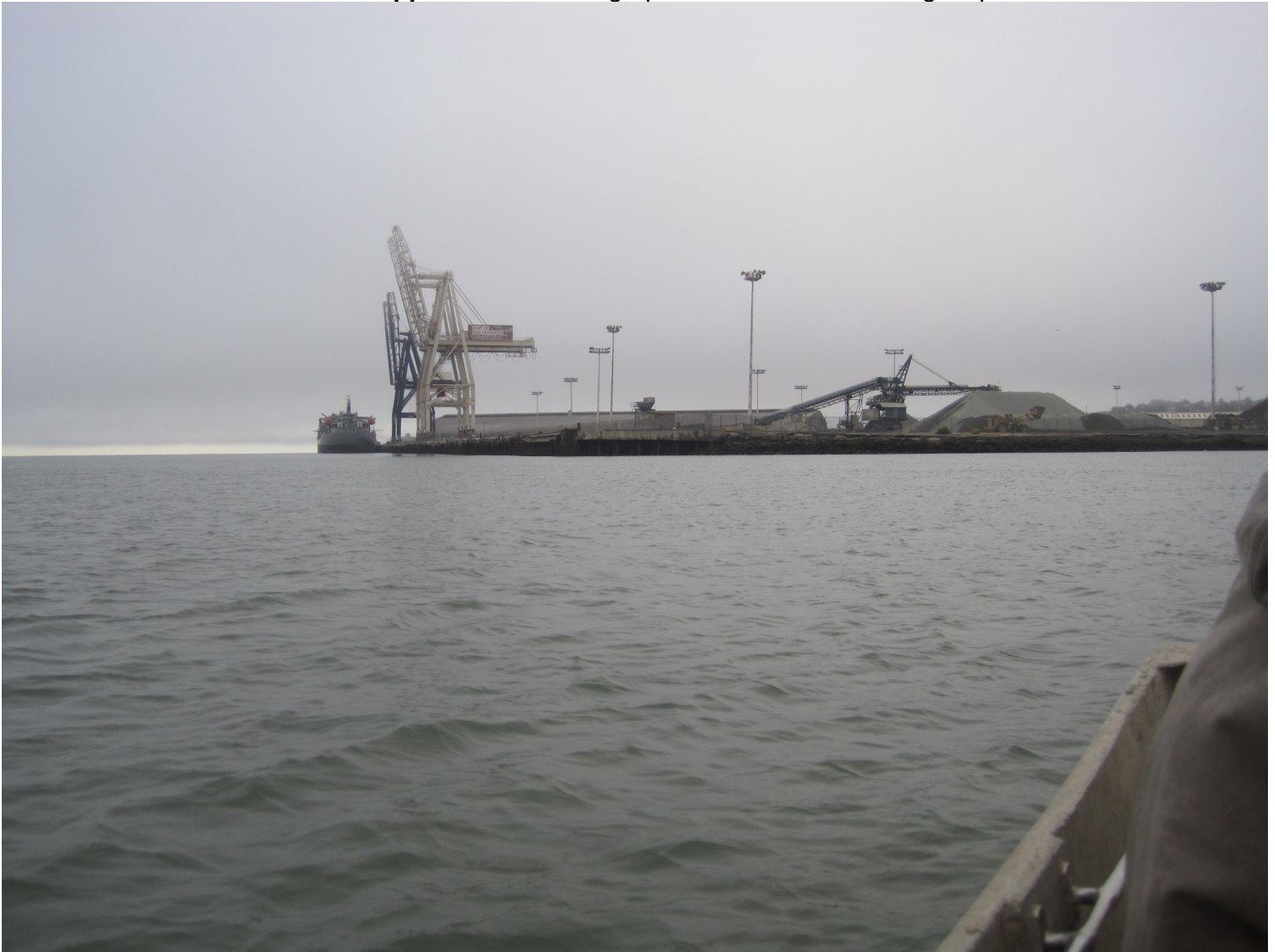
Photo 1. Overall view looking at north-east
