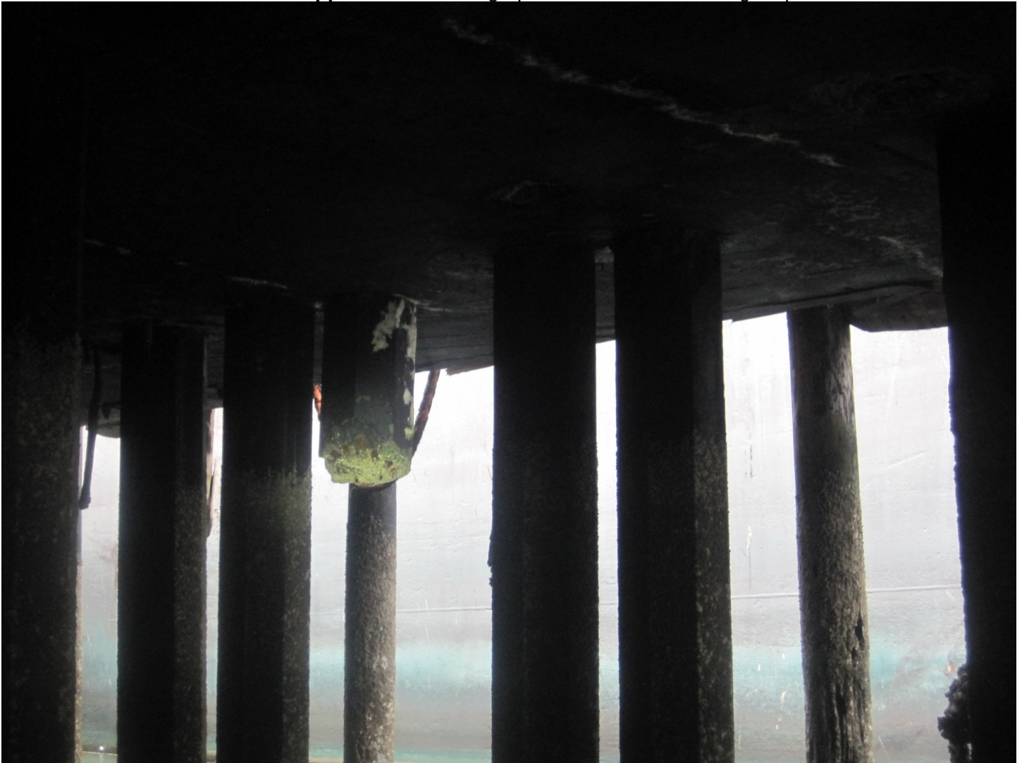
Photo 5. Missing pile
